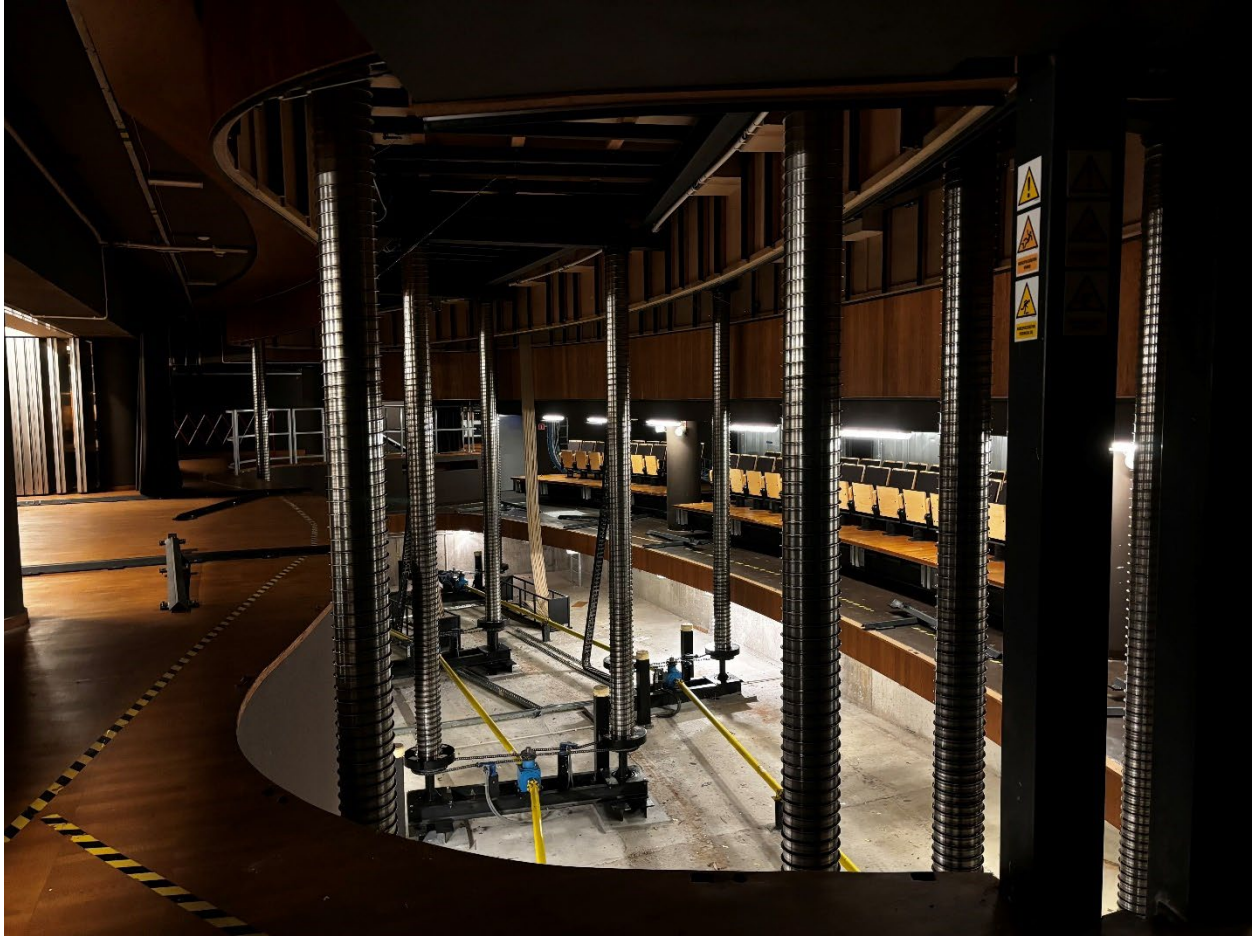
Fig. 12. Kuryłowicz and Associates, the lifts that elevate sections of the stage and isolate it from the surrounding structure, National Forum of Music, Wrocław, Poland, 2024.
