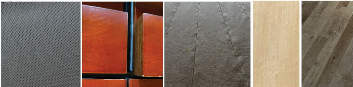
Fig. 12. Kimmo Lintula and Hannu Tikka, Sibelius Hall materials details from left to right textured wood acoustic paneling behind the stage, acoustic red wood panels, acoustic curtains, wall wood panels, and stage wood, Sibeliustalo, Lahti, Finland, 2024.
