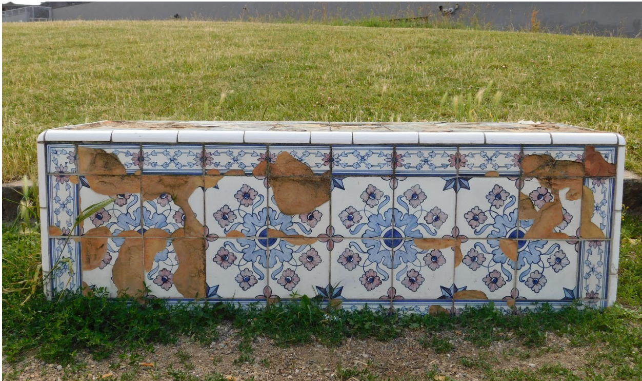
Figure 5: A bench from Portugal in Superkilen, whose tiles fell due to environmental conditions, not vandalism Source: Author
