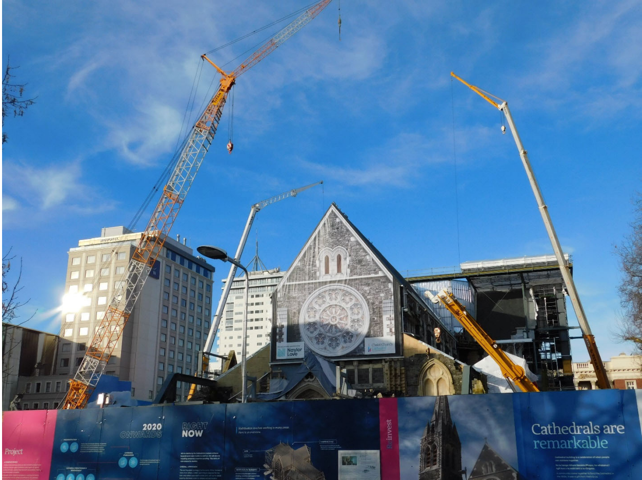
Figure 3: Image of Christchurch Cathedral under restoration present day Source: Author
