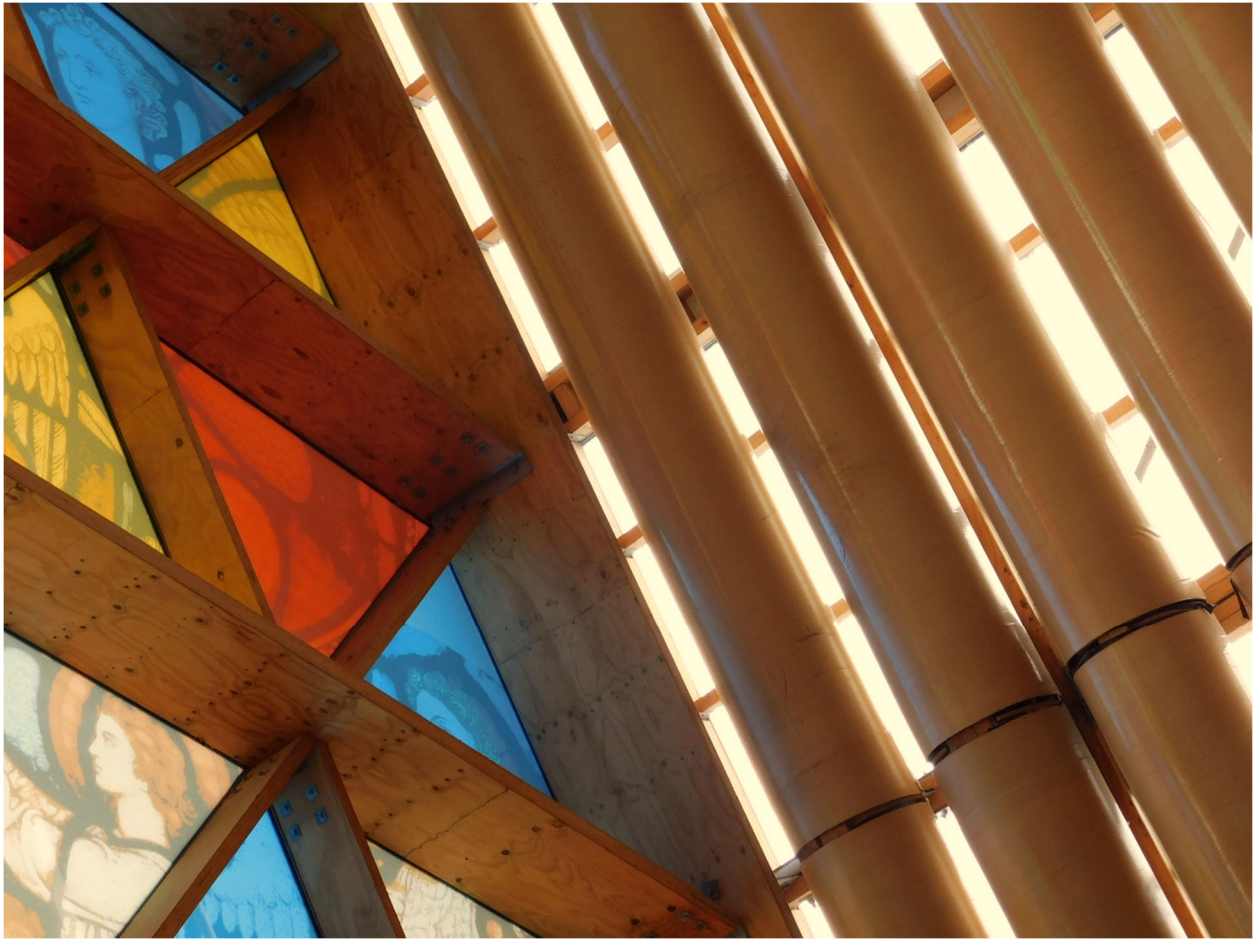
Figure 4: Interior Image of Transitional Cathedral in Christchurch, New Zealand, demonstration of cardboard construction and stained-glass motif. Source: Author
