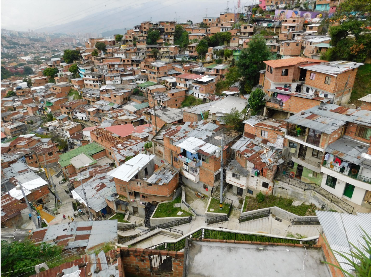
Figure 1: Public park infrastructure incorporated into Comuna 13, Medellín, Colombia Source: Author
