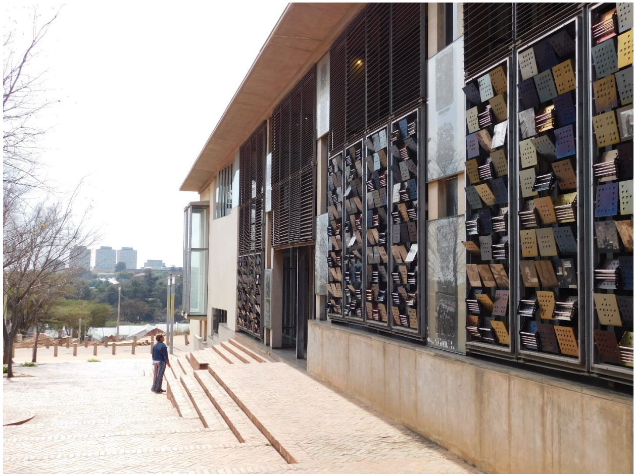
Figure 29: Image of the Great African Steps and western façade of gallery and sunscreens.
