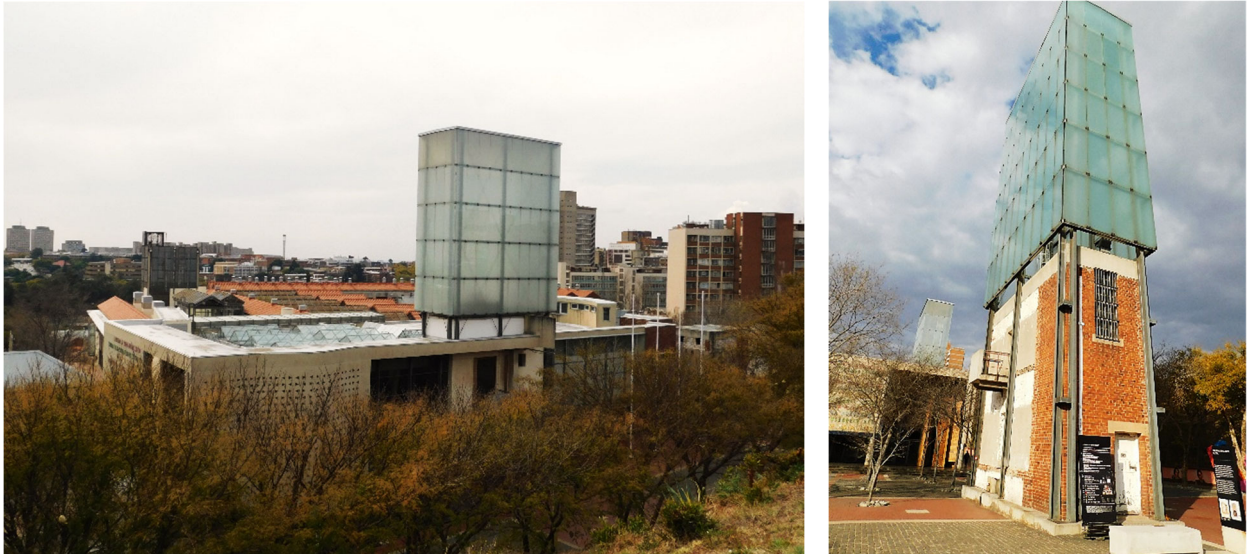
Figure 20(left) and 21(right): Images of the preserved trial block stairwells and lanterns installed on top
