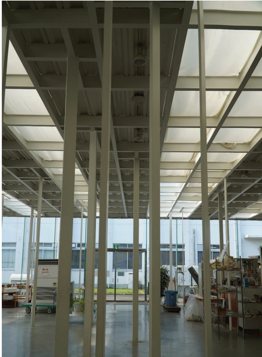
Figure 3: Junya Ishigami, view from inside of workshop showing varying column profile sizes, Kanagawa Institute of Technology Workshop, Kanagawa, Japan, July 15, 2023. Photo taken by author.
