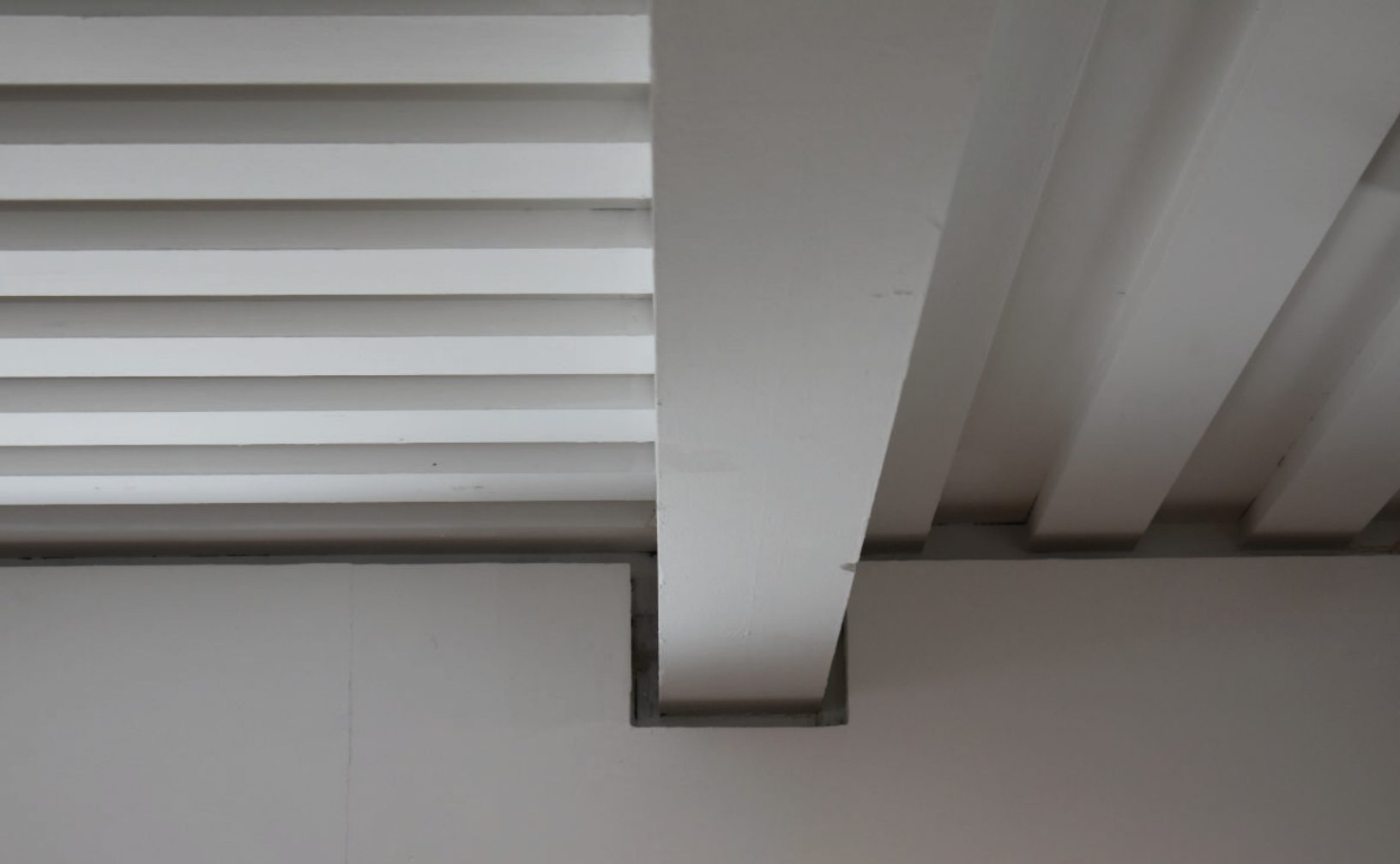
Fig. 82 natural light washing over structural members and ceiling
