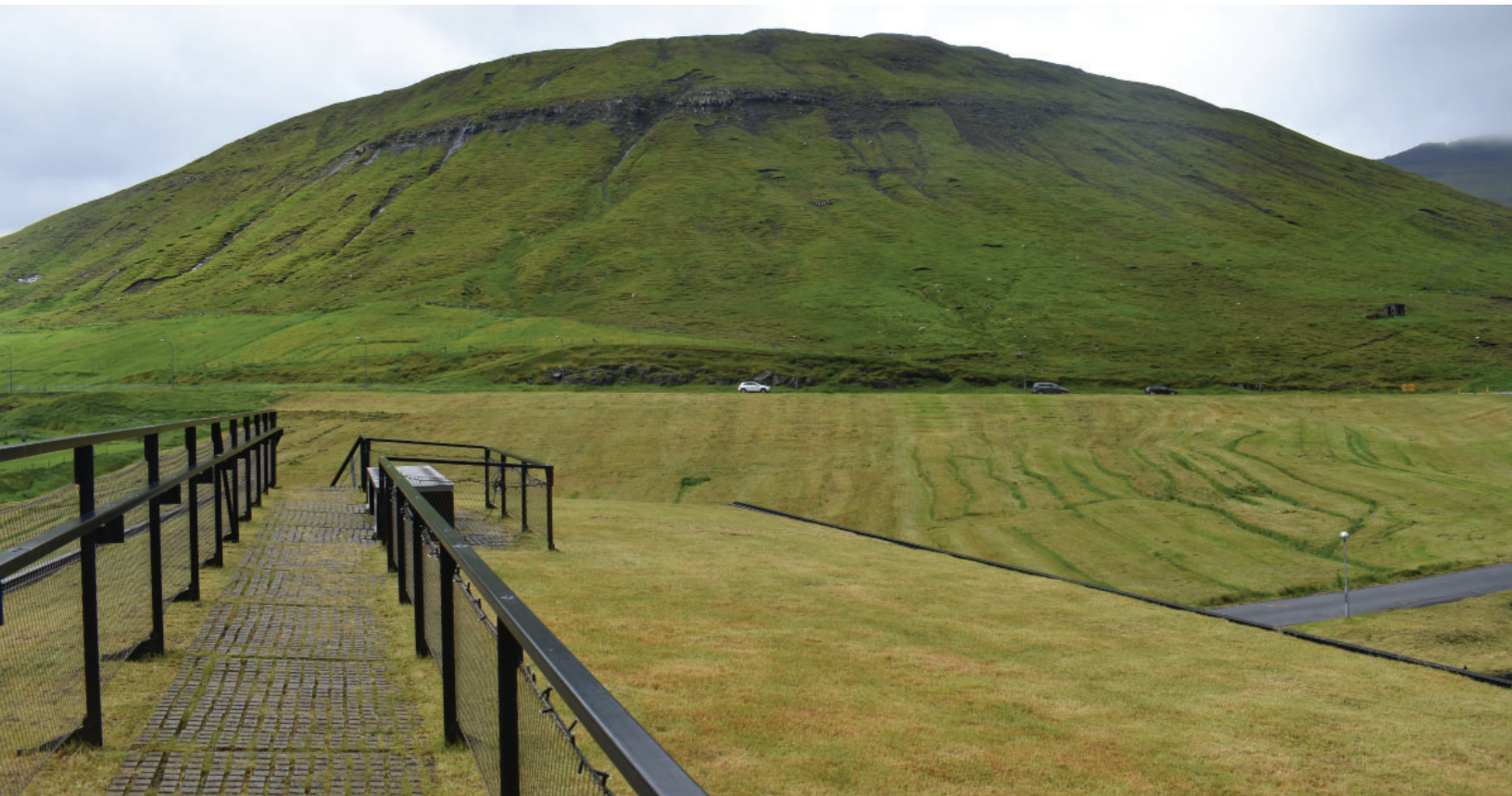
Fig. 13 view to the south-east displaying the building's landscape-like qualities
