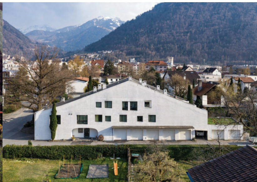
Fig. 75 Apartment building Urech Heroldstrasse 25, Chur | 1972 - 1973 photo courtesy of Ralph Feiner, Malans
