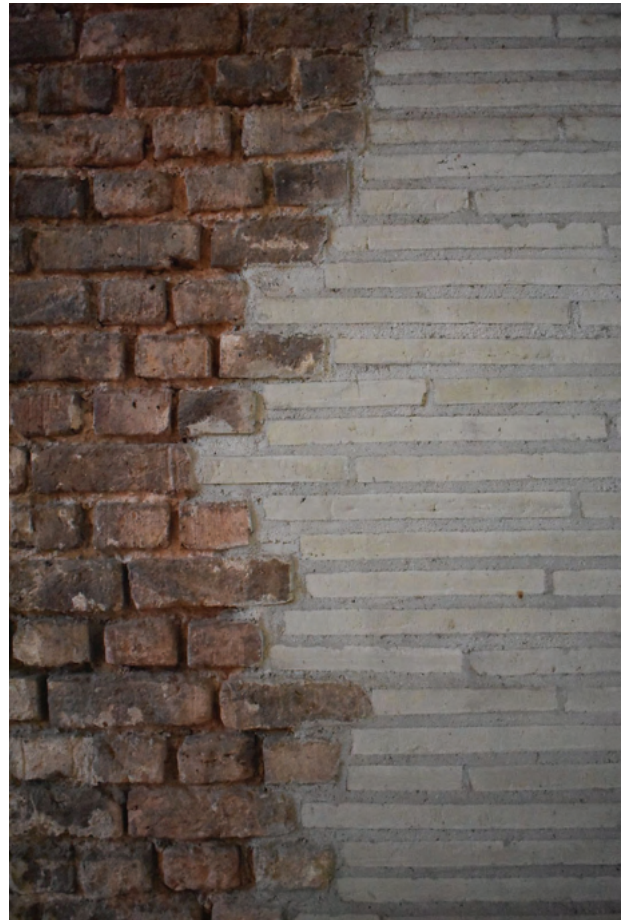
Fig. 43 old masonry walls sealed by new tiles
