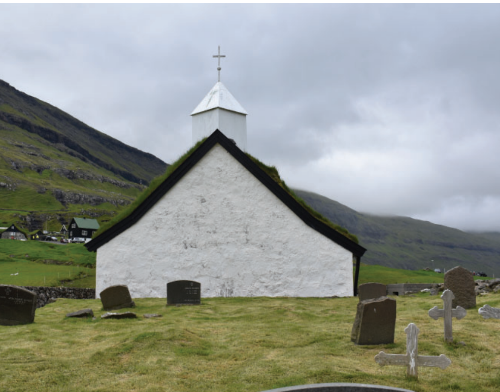
Fig. 04 & 05 old church in Saksun, Saksunar Kirka c. 1858, featuring turf roof construction
