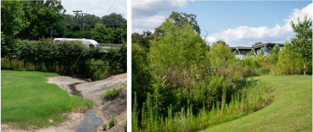
Fig. 9. Polluted stormwater drains across I-630 to the library.
