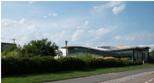
Fig. 8. View from Bremen Street Park.
