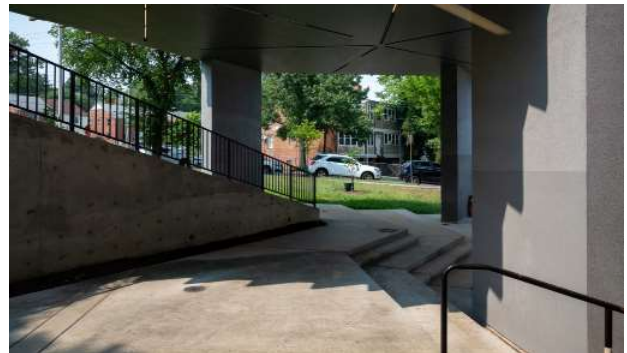
Fig. 7. View from interior to neighborhood.
