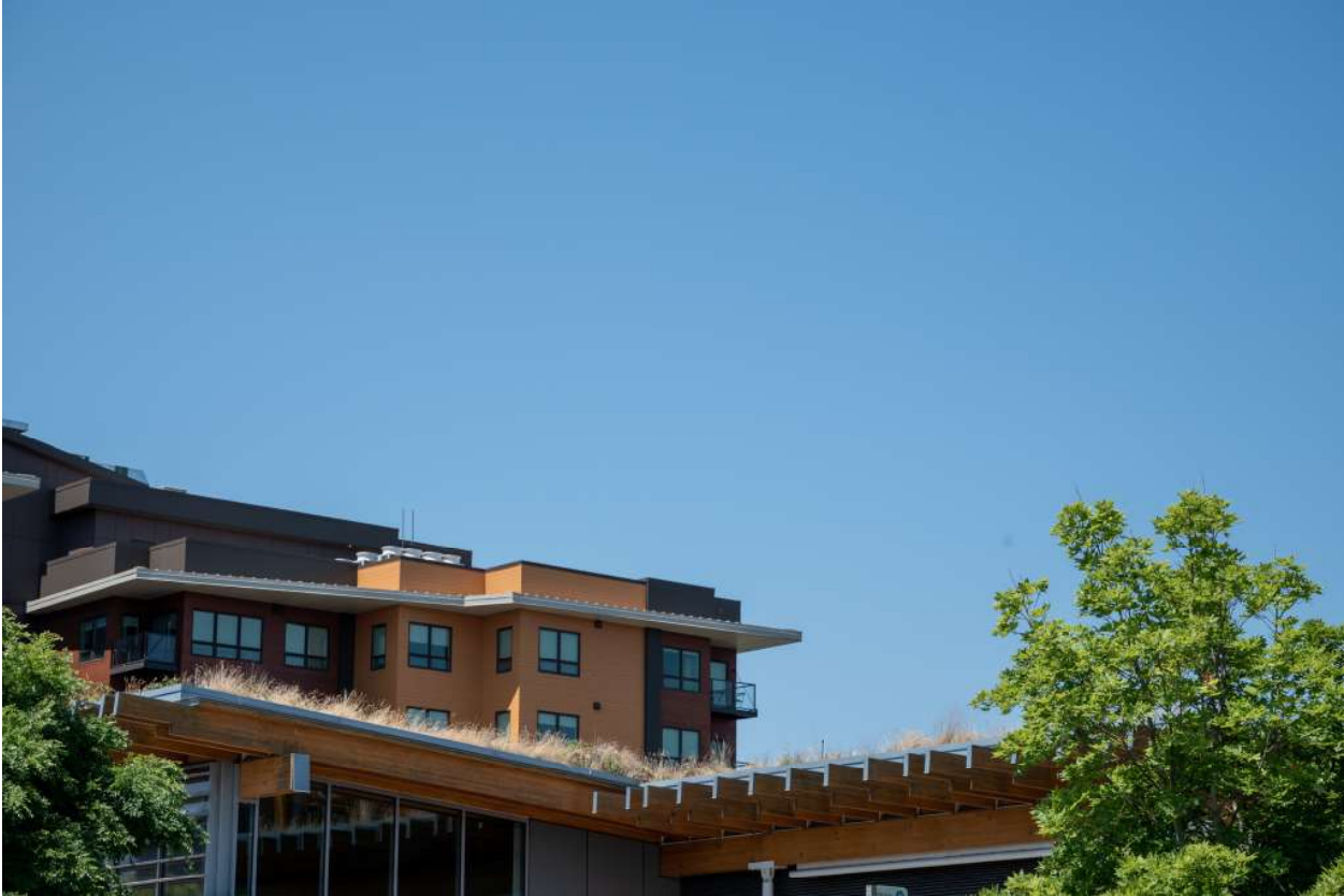
Fig. 5. Bohlin Cywinski Jackson, green roof and local housing, Ballard Branch Library, Seattle, WA, 2005.
