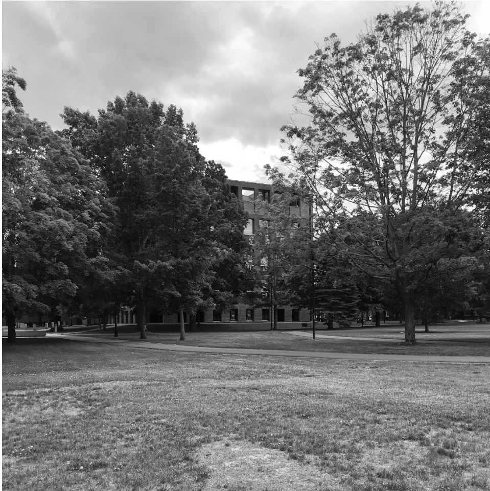
Figure 1: Louis I. Kahn. Northern elevation viewed from the lawn. Library at Phillips Exeter Academy, Exeter, NH, 1967-72.
