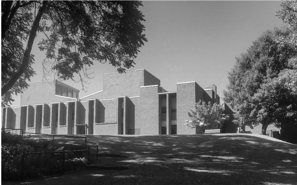
Figure 8: Louis I. Kahn. Southern façade viewed from the woodland area behind the church. First Unitarian of Rochester, Rochester, Ny, 1959-67.
