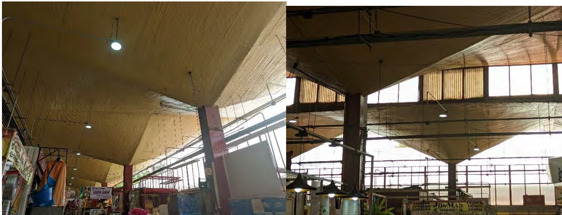
Fig.9. Felix Candela, View of interior structure, Mercado de Coyoacán, 1955.
