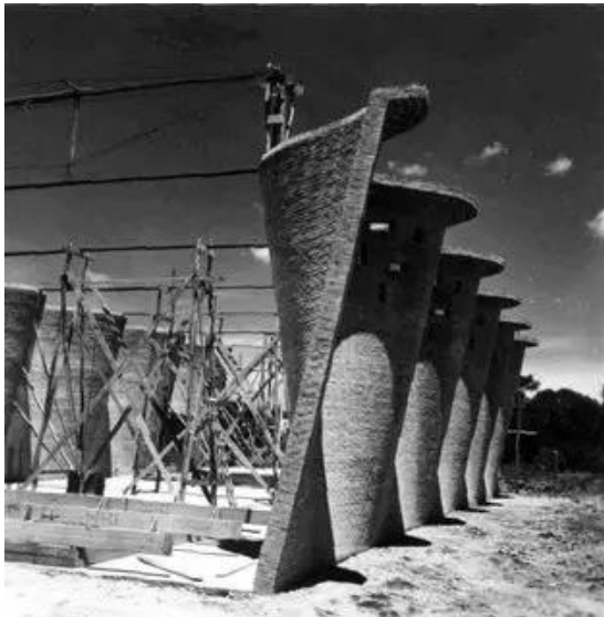
Fig. 12 Eladio Dieste, Photo of Construction, Cristo Obrero, Atlántida, Uruguay, 1953-60. 51
