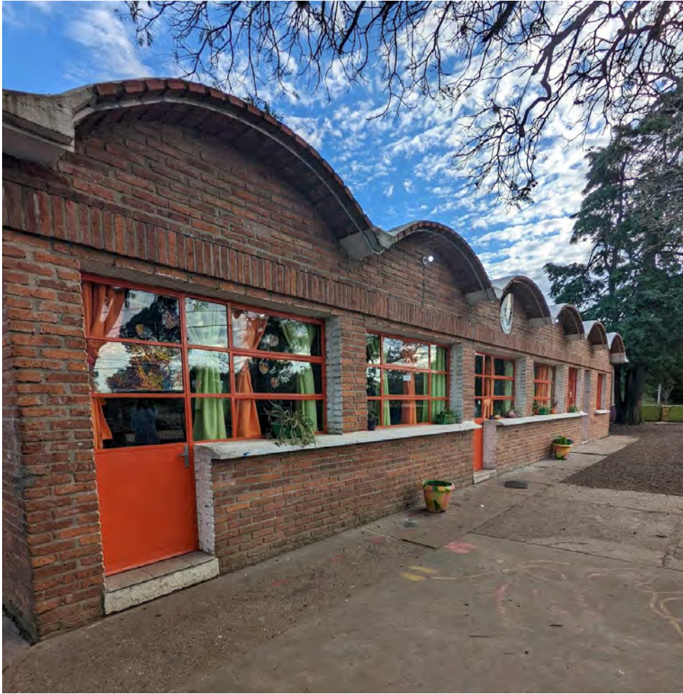
Fig.9 Eladio Dieste, View of classroom, Escuela rural tipo, Canelones, Uruguay, 1962-1975.
