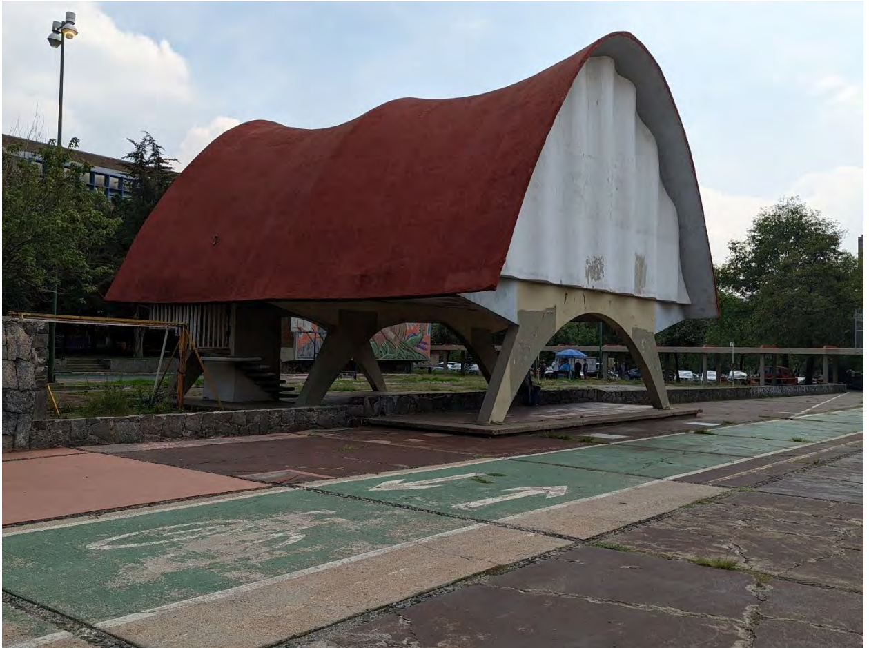
Fig. 7. Felix Candela, View of Exterior, Cosmic Ray Pavilion, Mexico City Mexico, 1951.
