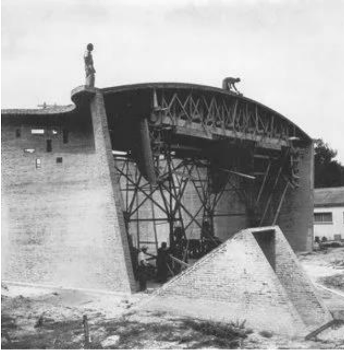
Fig. 13 Eladio Dieste, Photo of Construction, Cristo Obrero, Atlántida, Uruguay, 1953-60. 52
