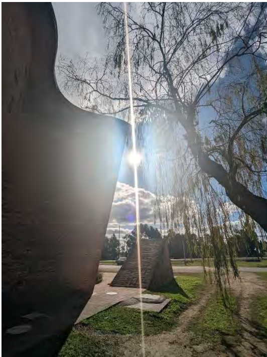
Fig.4. Eladio Dieste, View of baptistry from church yard,, Cristo Obrero, Atlántida, Uruguay, 1953-60.
