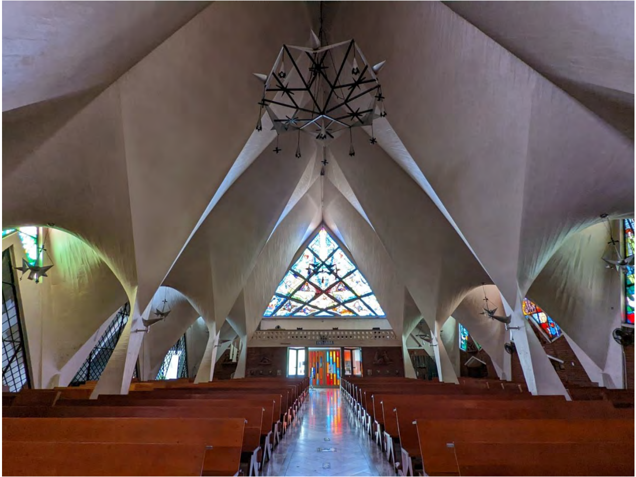
Fig. 1. Felix Candela, Interior view of main entrance to main nave and alter, La Medalla Milagrosa, Mexico City, Mexico, 1953-1957.
