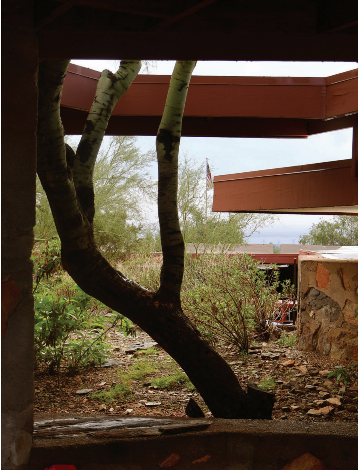
Fig. 01. Frank Lloyd Wright, roof detail, Taliesin West, Scottsdale, Arizona, USA, October 2025
