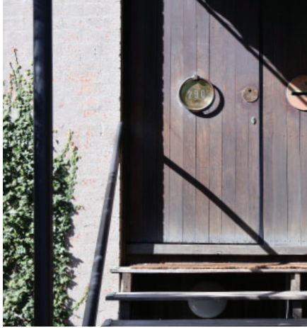
Fig. 03. Robin Boyd, front entrance, Boyd's House II, Melbourne, VIC, Australia, August 2025
