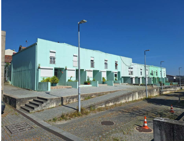
Fig. 2. Alvaro Siza Vieira, Sao Victor Housing, Porto, Portugal, 1974. (Photo by Author)
