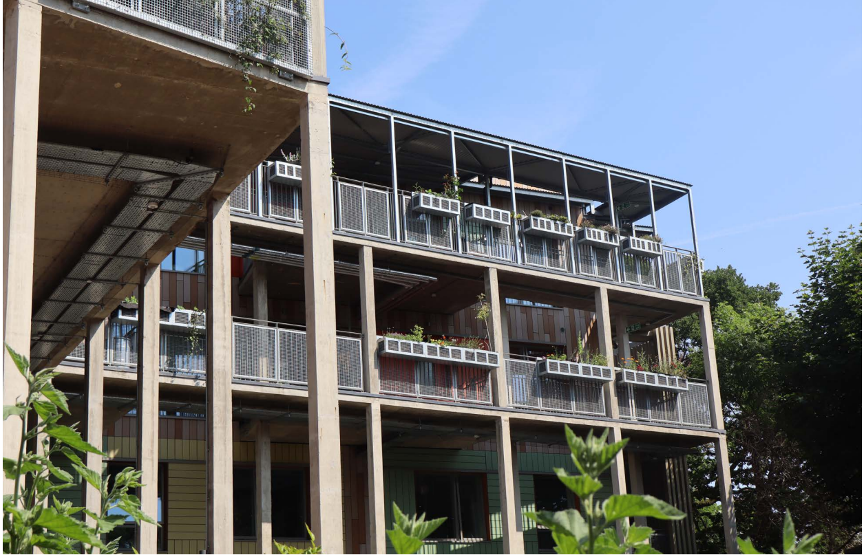
Fig. 18. Jon Broome, The Rural Urban Synthesis Society, A New Take on Co-op Housing, London, UK, 2025. (Photo by Author)
