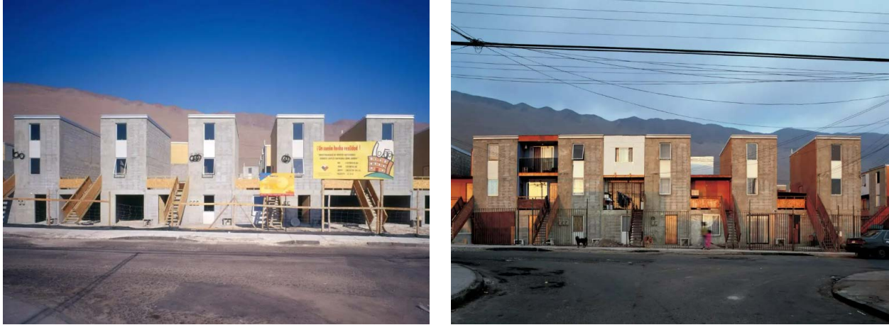
Fig. 8. Alejandro Aravena, Quinta Monroy Before and After Expansions, Iquique, Chile, 2003. Source: Elemental Arquitectos
