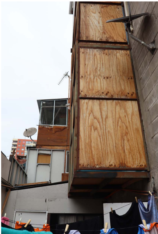
Fig. 10. Illegal Expansions Such as Cantilevers or a Third Floor, Quinta Monroy, Chile, 2025. (Photos by Author)
