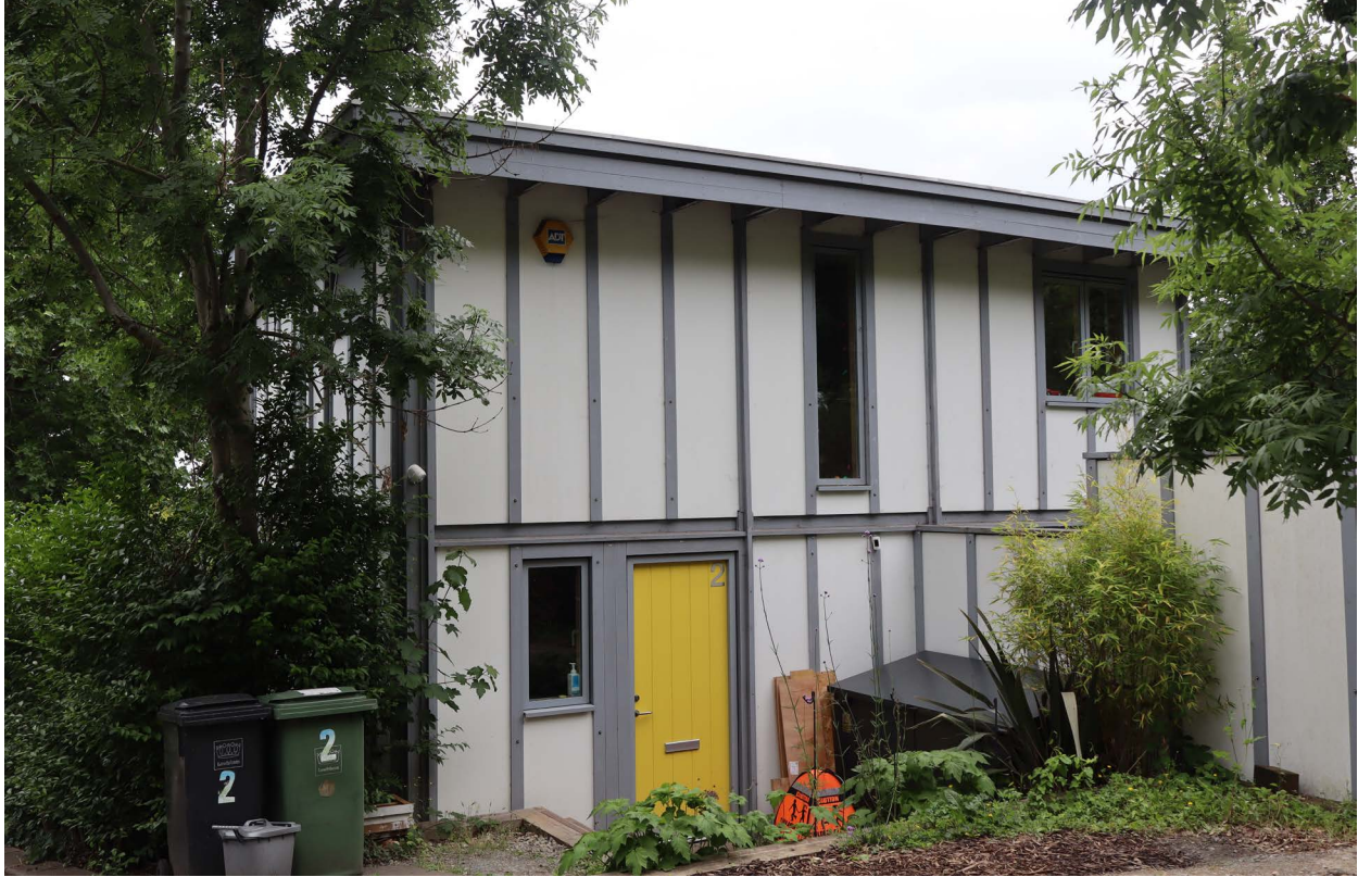
Fig. 14. Walter Segal, House in Walter's Way, London, UK, 2025. (Photo by Author)
