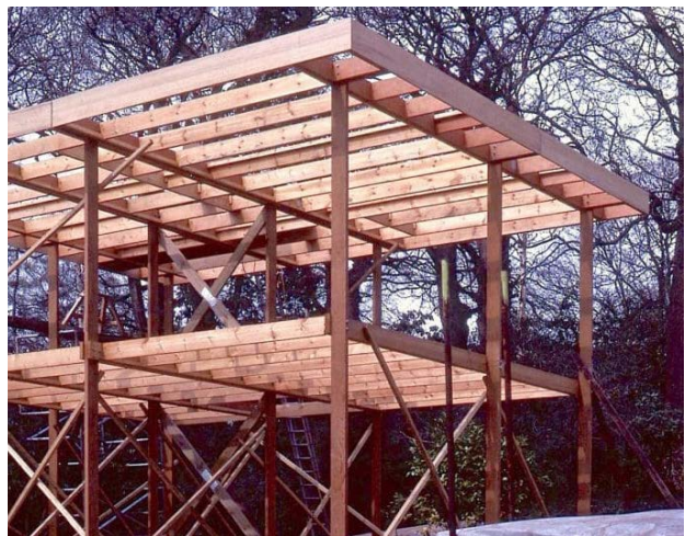
Fig. 6. Walter Segal, Columns and Floors Erected , London, UK, 1979. Source: drawingmatter.org
