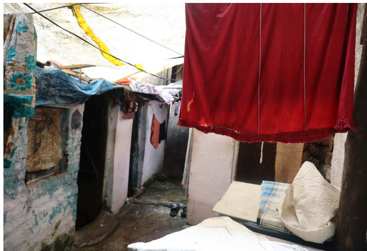
Fig. 3. A Kuchha (unsafe) House, Yerwada, Pune, India, 2025. (Photo by Author)
