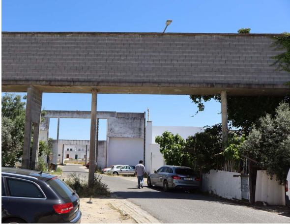
Fig. 13. Infrastructural Conduit Provides Necessary Urban Scale, Malagueira, Portugal, 2025. (Photo by Author)
