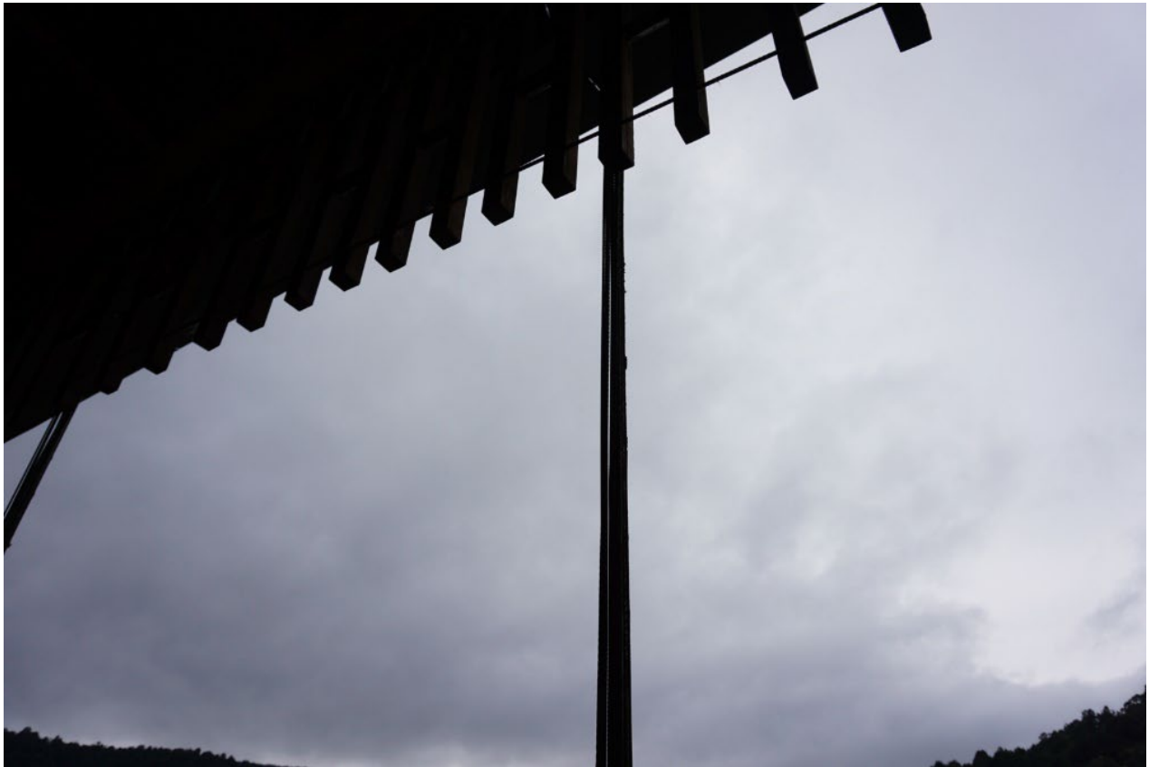
Figure 14: Water Collecting Steel Cables
