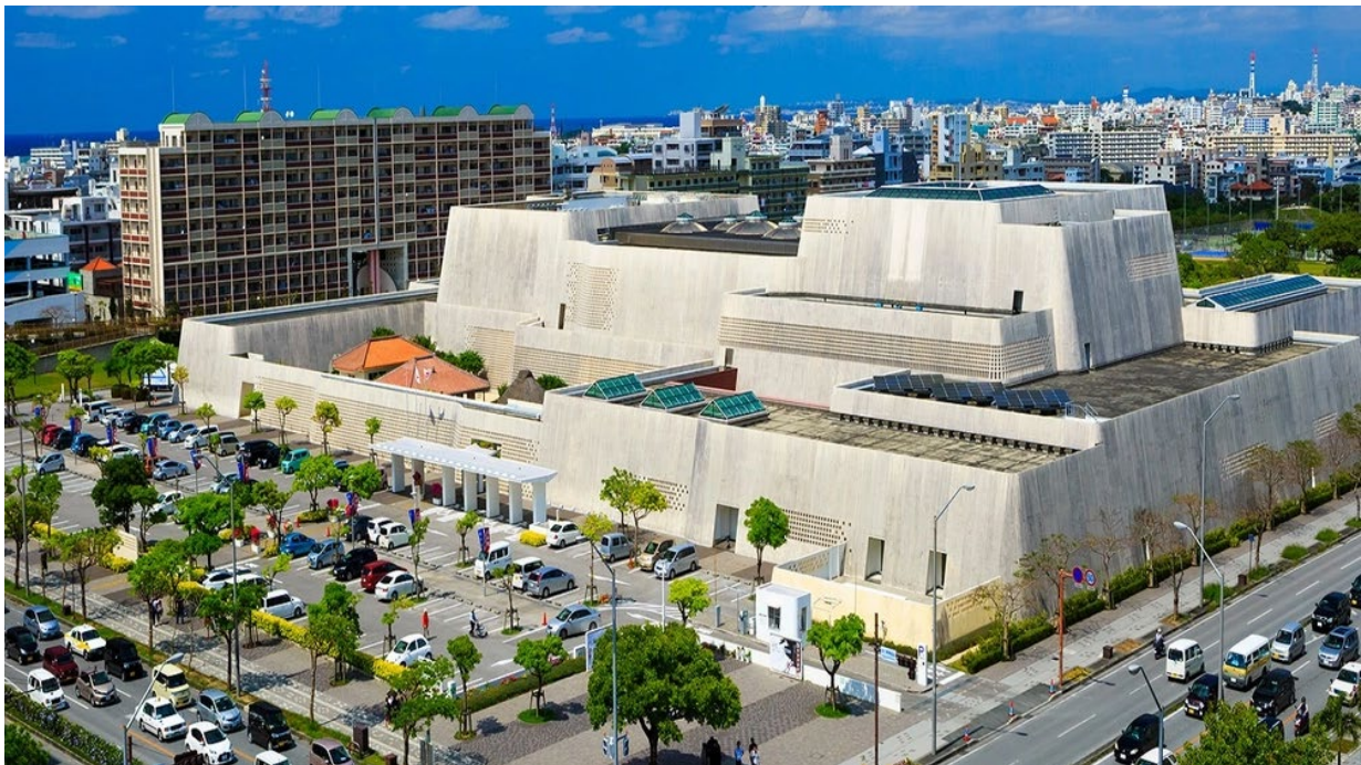
Figure 12: Okinawa Prefectural Museum Exterior View. Source: Traveloka
