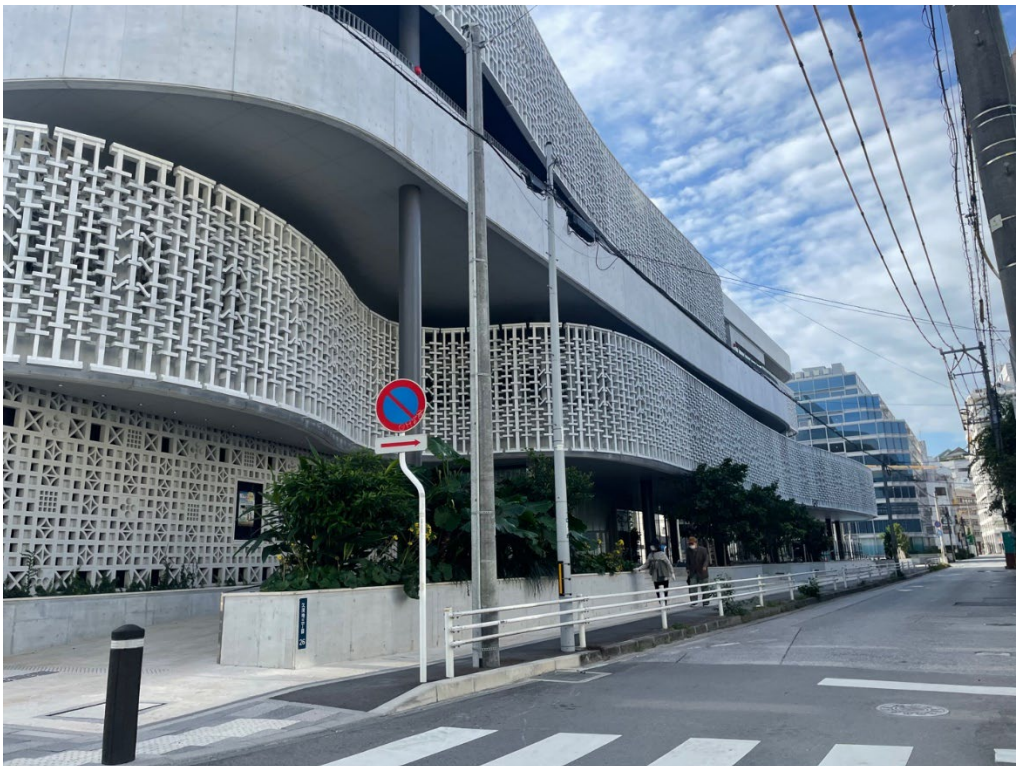
Figure 21: Building Utilizing Hana Blocks (2023)
