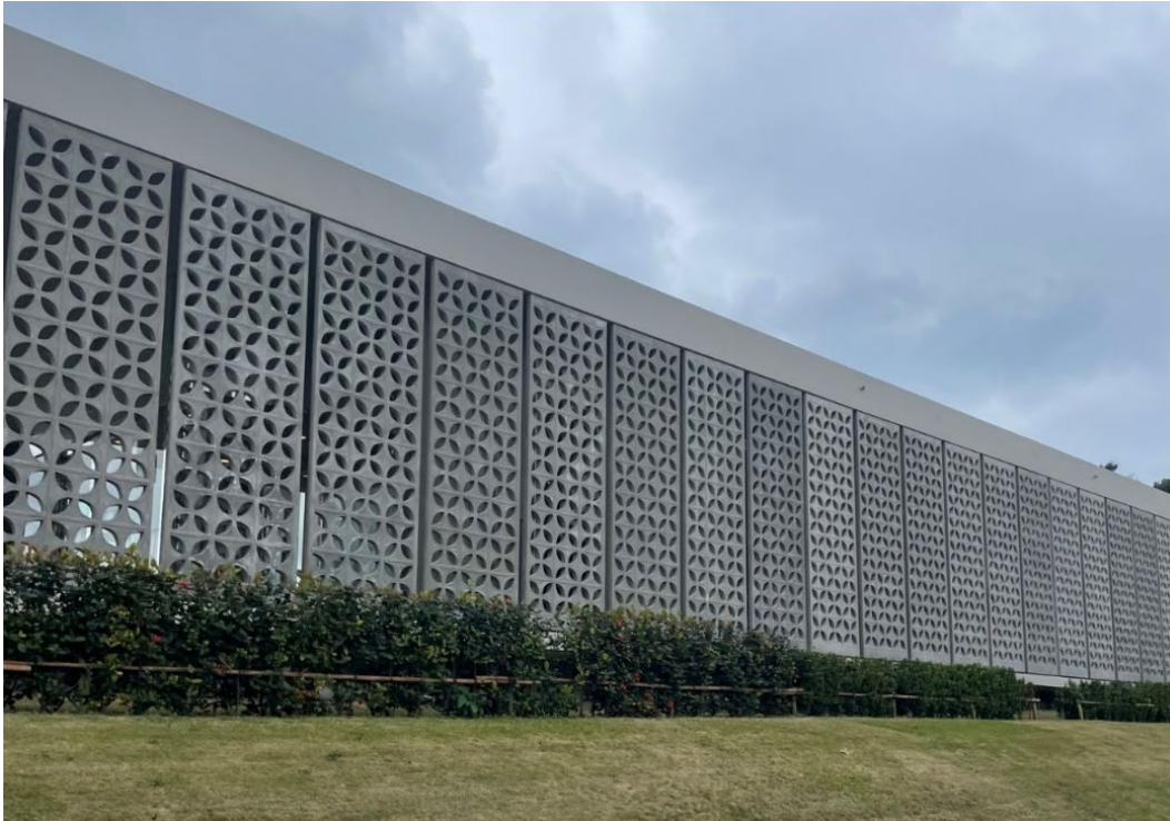
Figure 22: Building Utilizing Hana Blocks (2024)
