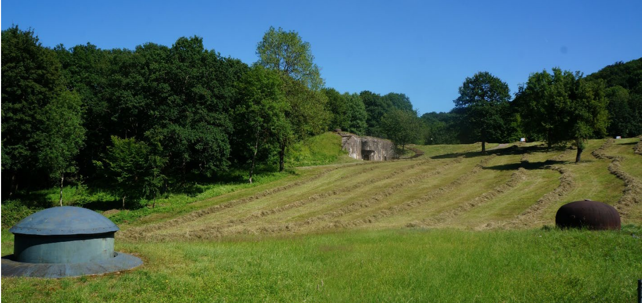
Fig. 5. Paul Painleve & C.O.R.F., view showing an artillery turret (left), infantry cloche (right), and fixed artillery block (center), Ouvrage Hackenberg, Vekring, France, 1929-1932.
