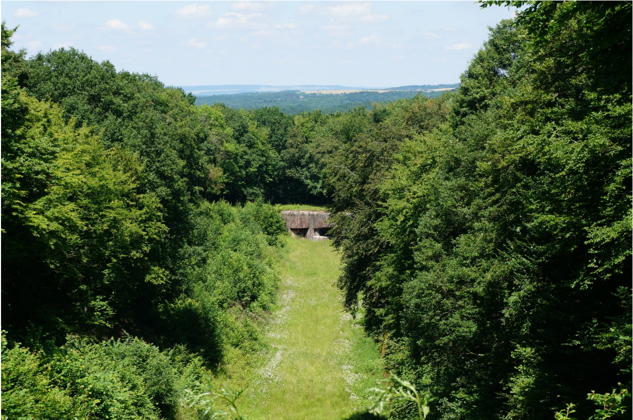
Fig. 15. Paul Painleve & C.O.R.F., overgrown anti-tank trench between Blocks 24 and 25 with Germany in the distance, Ouvrage Hackenberg , Vekring, France, 1929-1932.
