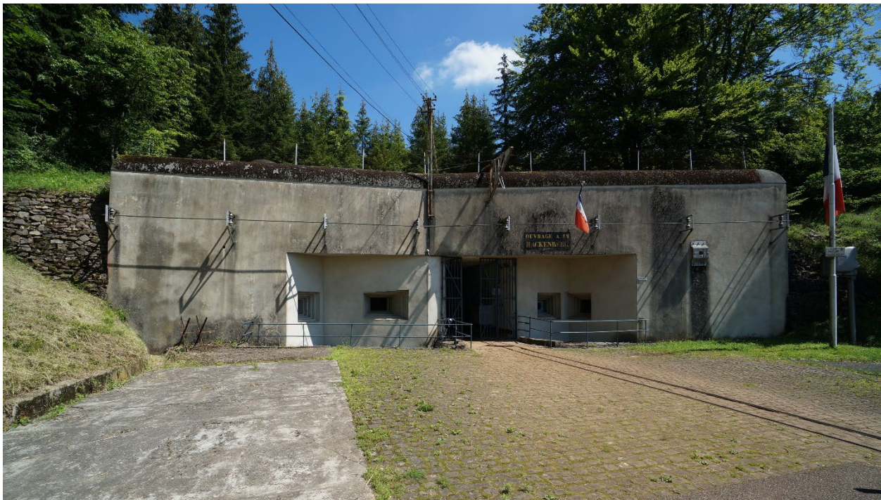
Fig. 6. Paul Painleve & C.O.R.F., view of Ouvrage Hackenberg's munitions entrance with rail gauge, electrical lines, and radio antenna at center, Ouvrage Hackenberg , Vekring, France, 1929-1932.
