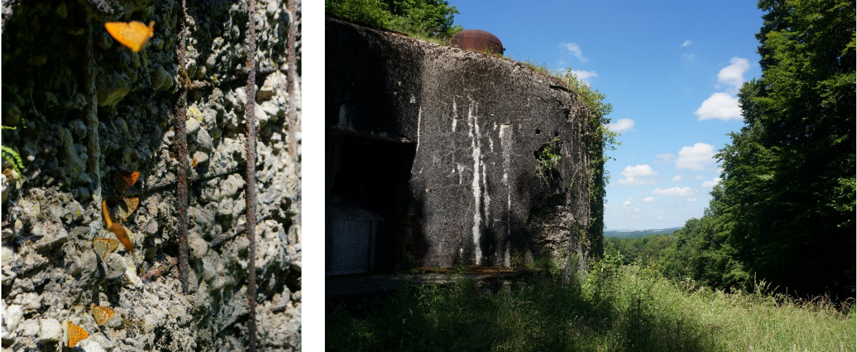
Fig. 18-19. Paul Painleve & C.O.R.F., butterflies inhabit reinforced concrete; Block 24 stands over an open border, Ouvrage Hackenberg , Vekring, France, 1929-1932.
