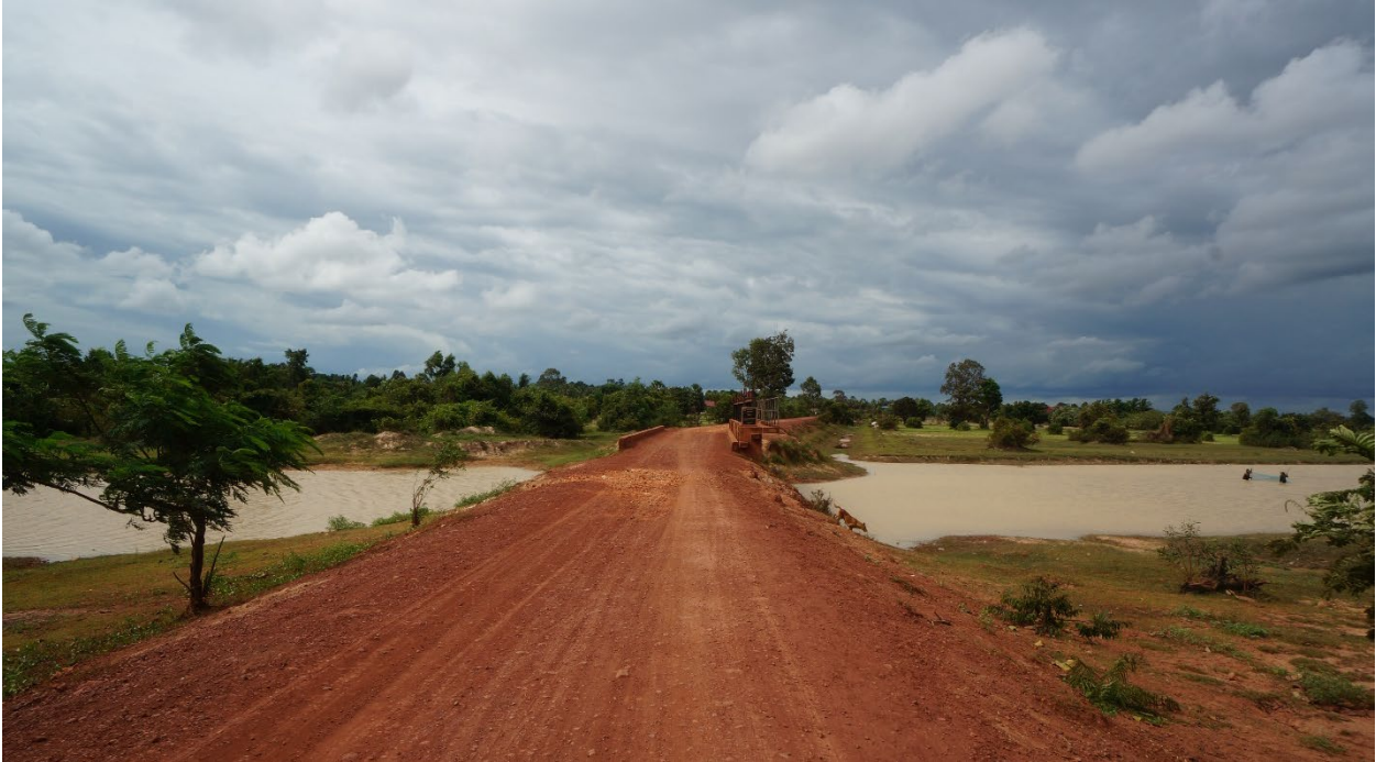
Fig. 16. A rural road and levee with a modern irrigation sluice doubles as both transportation and agricultural infrastructure, Angkor Archaeological Park, Cambodia.
