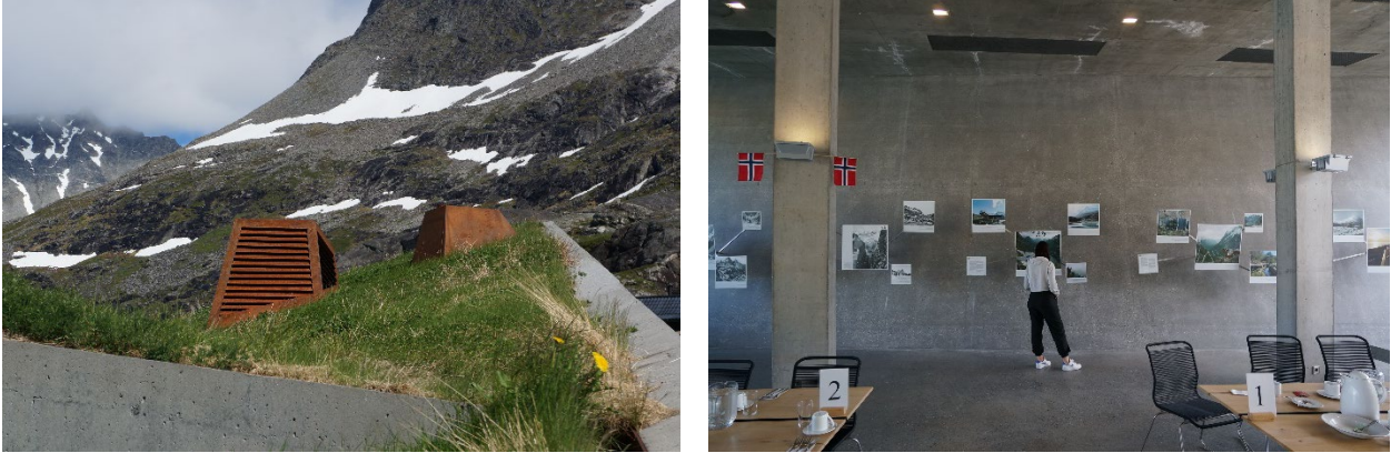
Fig. 6-7. Reiulf Ramstad Arkitekter, vernacular and highly insulative sod roofs with HVAC and kitchen exhaust ducts; a visitor inspects the gallery, Norway, 2005-2012.
