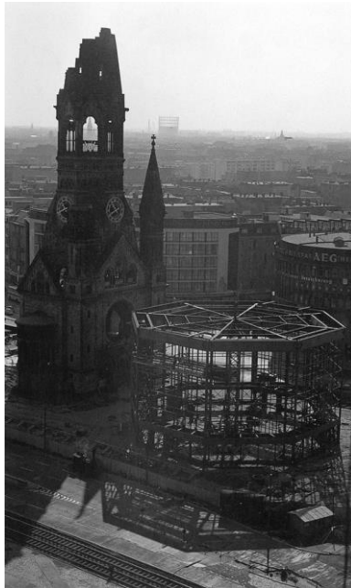
Fig. 14 Egon Eiermann, structure of the new church during construction, Kaiser Wilhelm Memorial Church, Berlin, Germany, 1959-63. Photo from Artstor
