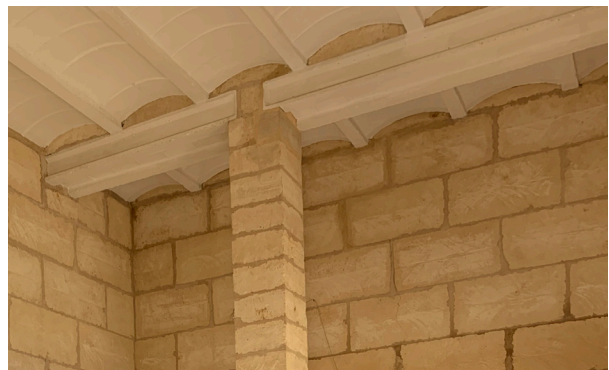
Fig. 24 - Sigurd Lewerentz, double beams and vaulted ceiling, St. Peter's Church in Klippan, 1963-66
