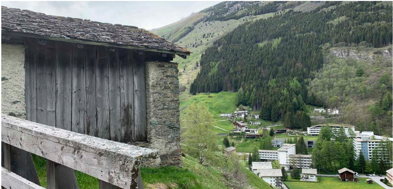
Fig. 8 - Wooden In-filled Opening of Farm Hut and Therme Vals Across the Valley with Similar Opening Source: author
