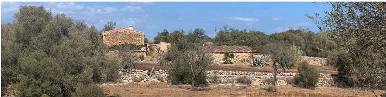
Fig. 35 - Multiple buildings of traditional rural Mallorcan house
