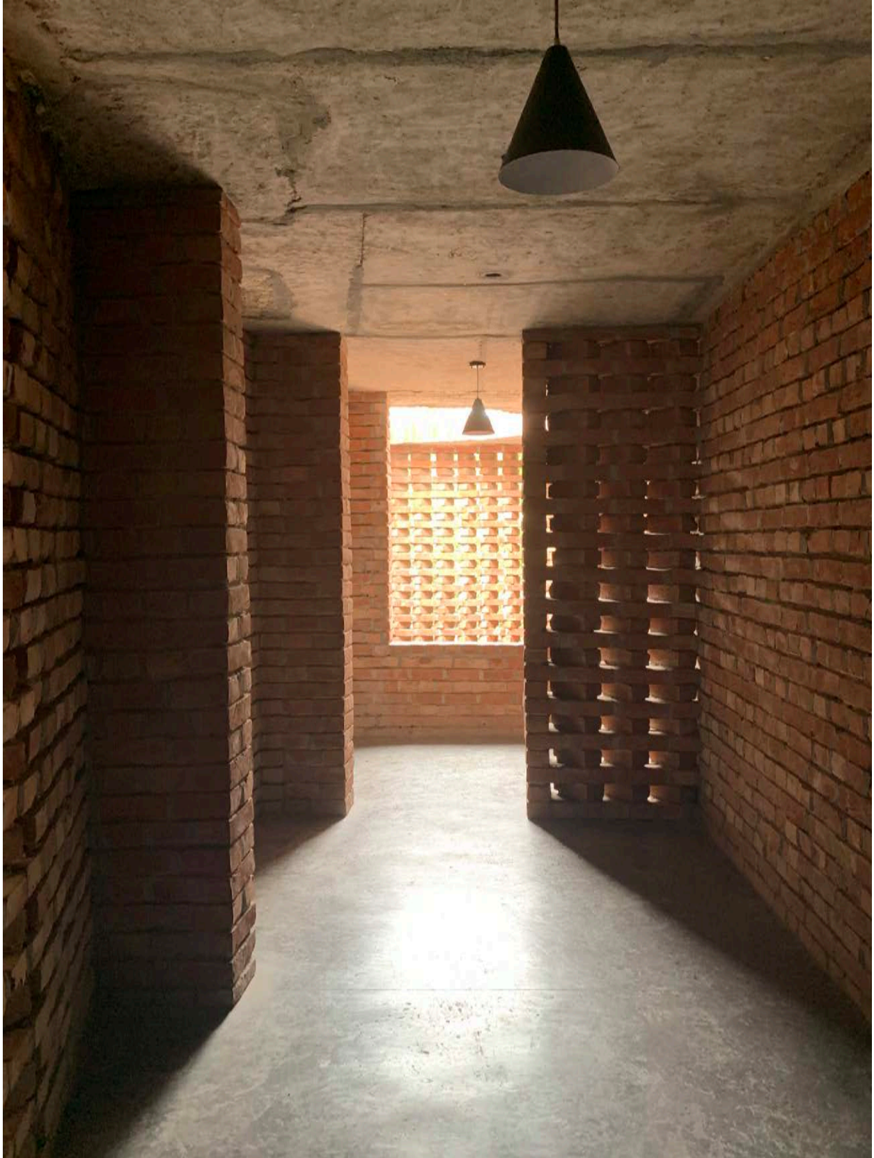
Fig. 17 - Marina Tabassum, interior view of second level hall of concrete and brick, Bait Ur Rouf Mosque, 2012 Source: author
