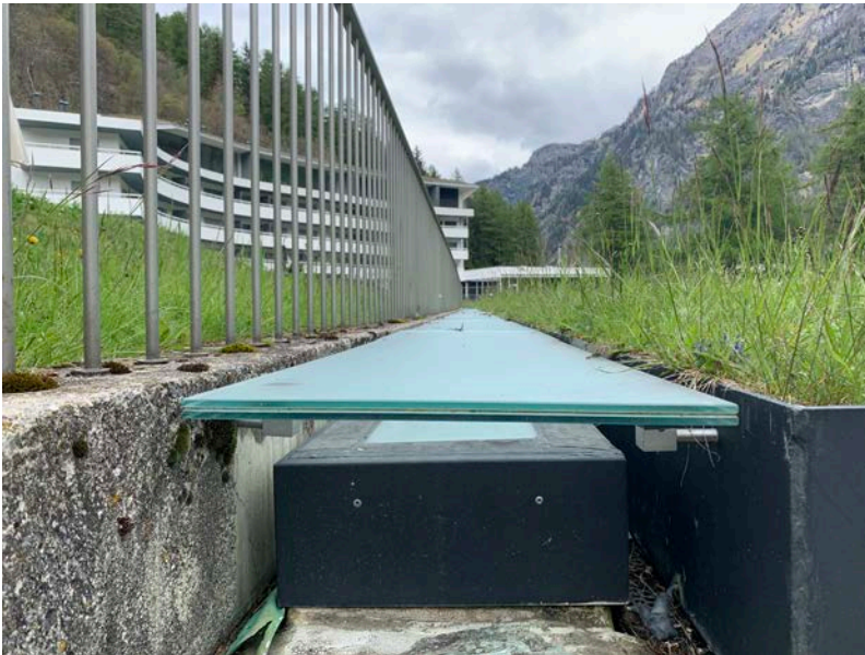
Fig. 13 - Peter Zumthor, ceiling reveal and expansion joint detail from exterior, Therme Vals, 1996
