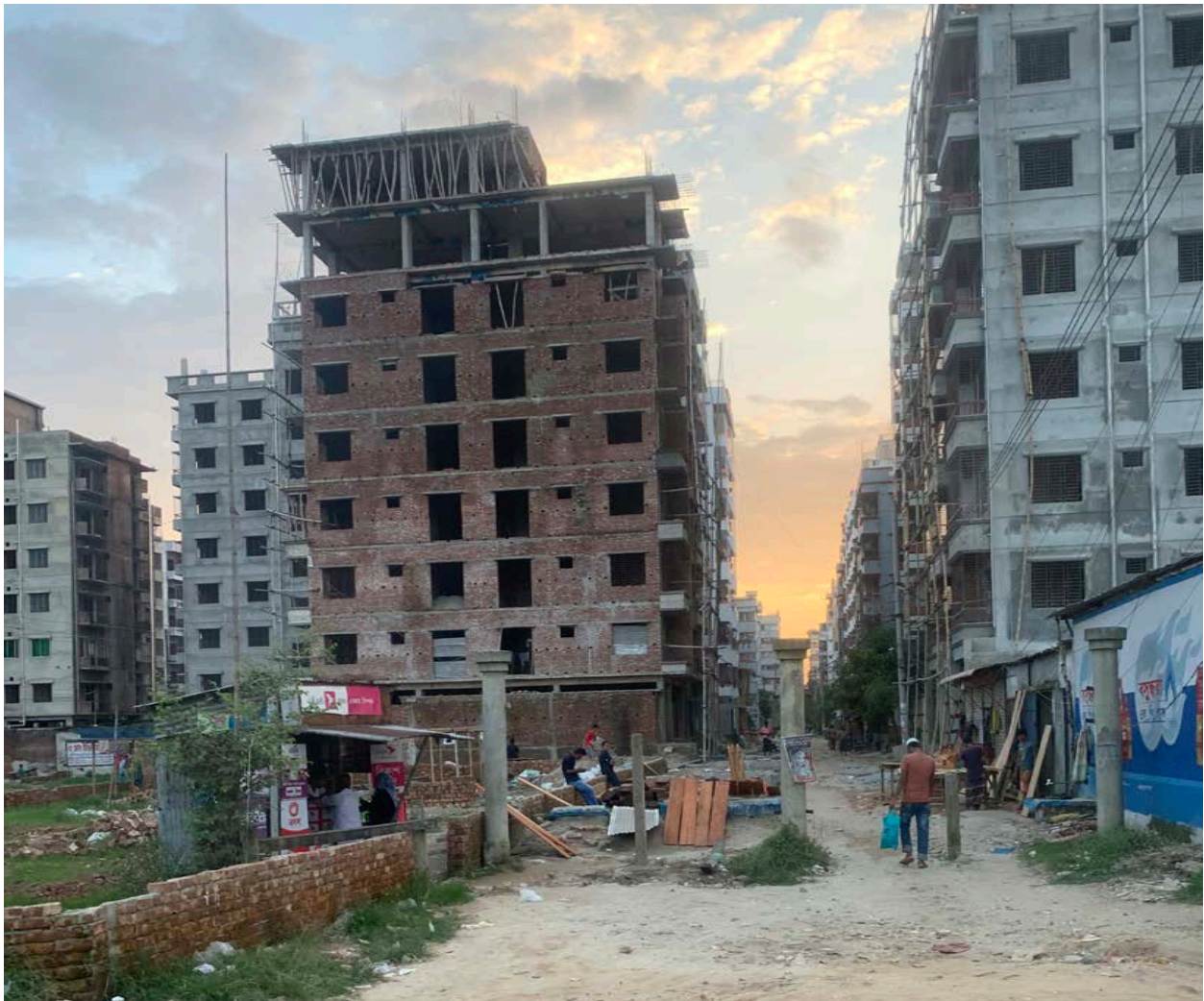
Fig. 12 - standard construction in Dhaka Source: author
