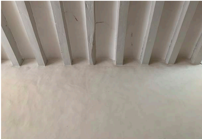
Fig. 14 - Bovedilla ceiling in traditional Mallorcan house Fig. 15 - Jørn Utzon, bovedilla ceiling in the entry porch, Can Lis Source: author
