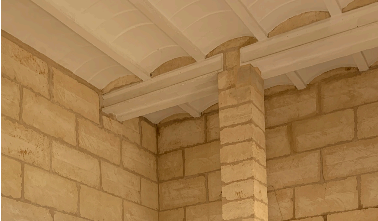
Fig. 12 - Jørn Utzon, structural system of load-bearing stone, concrete columns, and bovedilla vaults, Can Lis, 1971 Source: author
