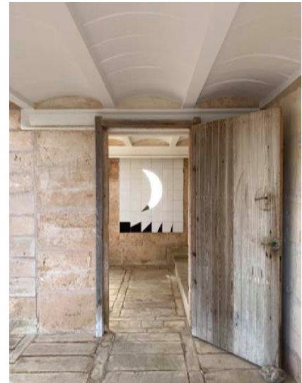
Fig. 14 - Bovedilla ceiling in traditional Mallorcan house Fig. 15 - Jørn Utzon, bovedilla ceiling in the entry porch, Can Lis Source: author
