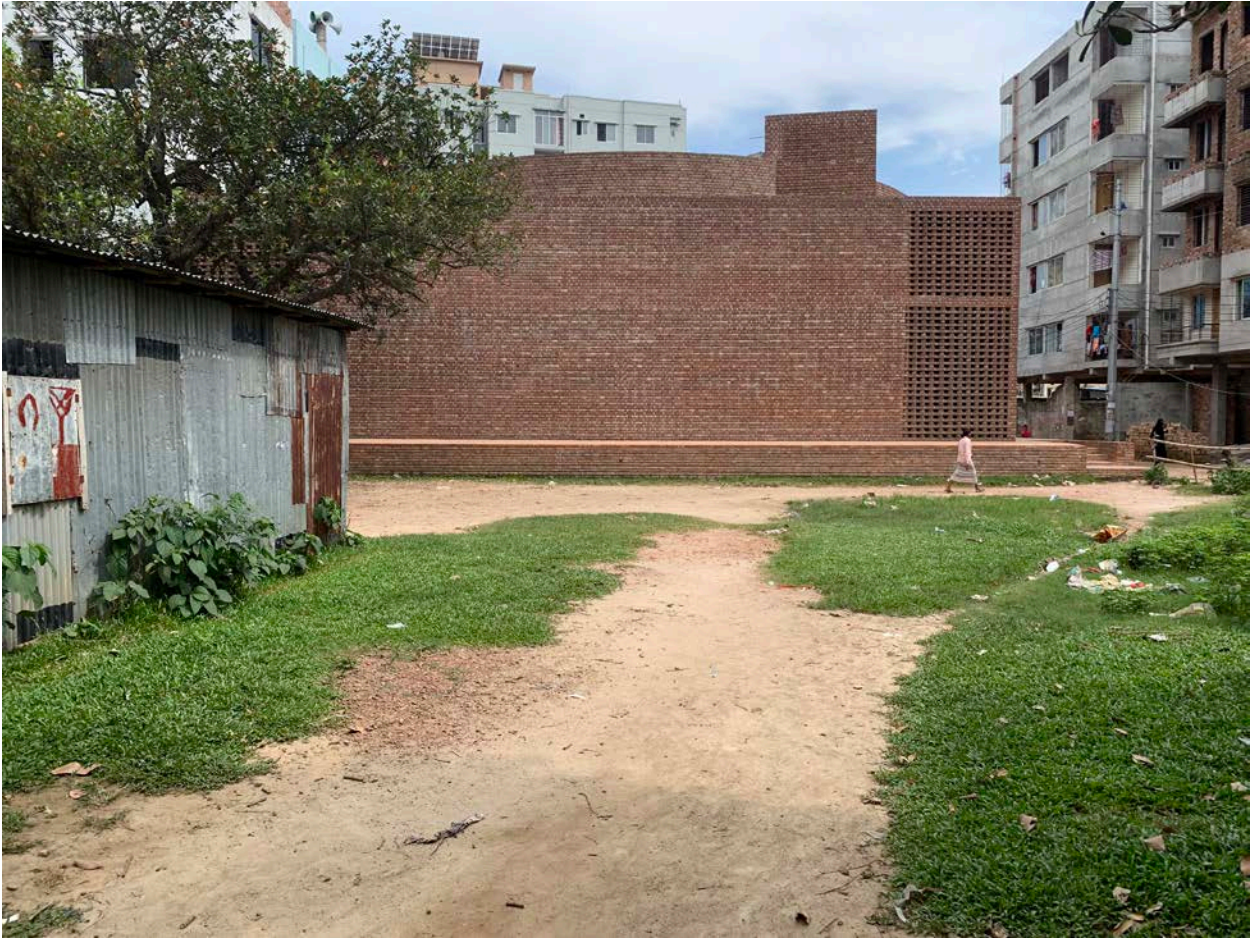
Fig. 32 - Marina Tabassum, exterior view from the north with jackfruit tree and tin-shed, Bait Ur Rouf Mosque, 2012 Source: author
