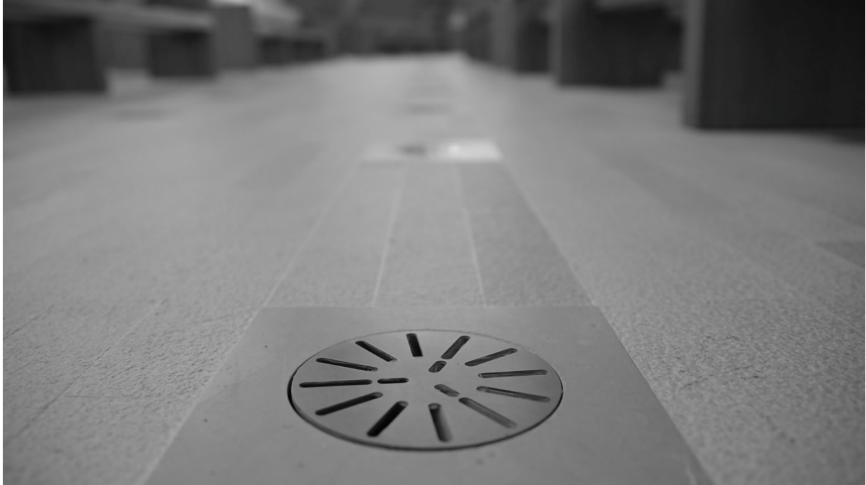
Fig. 11. Renzo Piano Building Workshop, view of interior drain where runoff water is collected, Padre Pio Pilgrimage Church, San Giovanni Rotondo, Italy, 2004 CE.
