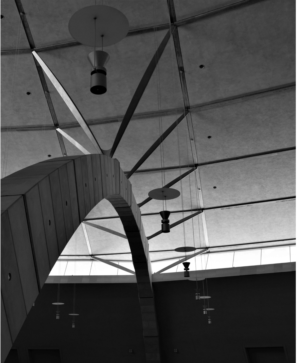
Fig. 12. Renzo Piano Building Workshop, view of arch with "V prop" and clerestory, Padre Pio Pilgrimage Church, San Giovanni Rotondo, Italy, 2004 CE.
