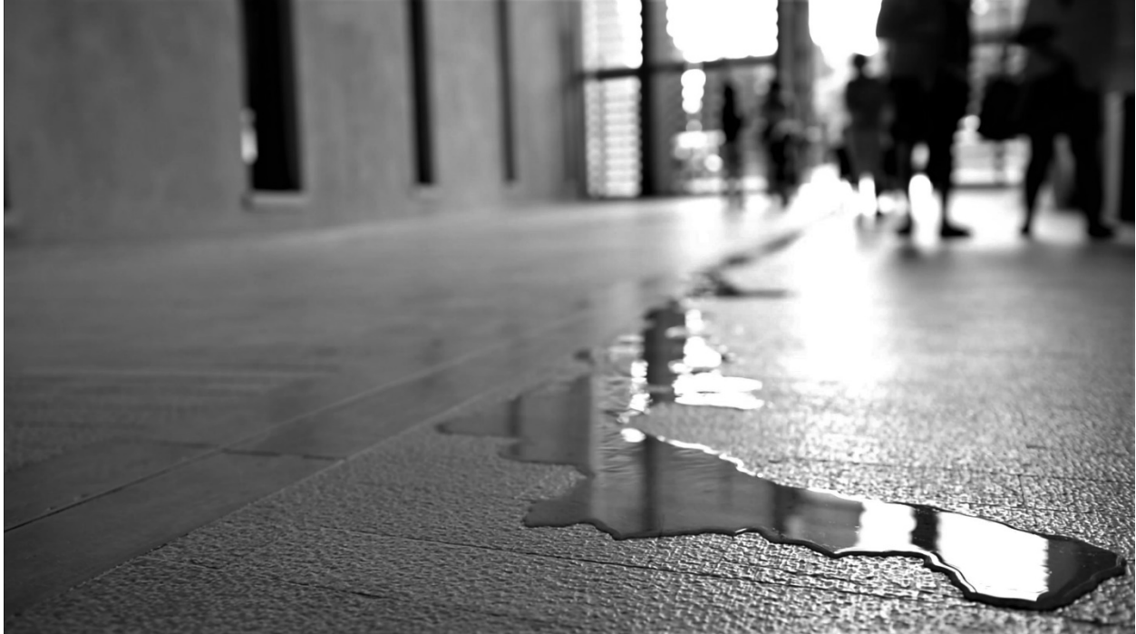
Fig. 10. Renzo Piano Building Workshop, view of water infiltrating sanctuary, Padre Pio Pilgrimage Church, San Giovanni Rotondo, Italy, 2004 CE.
