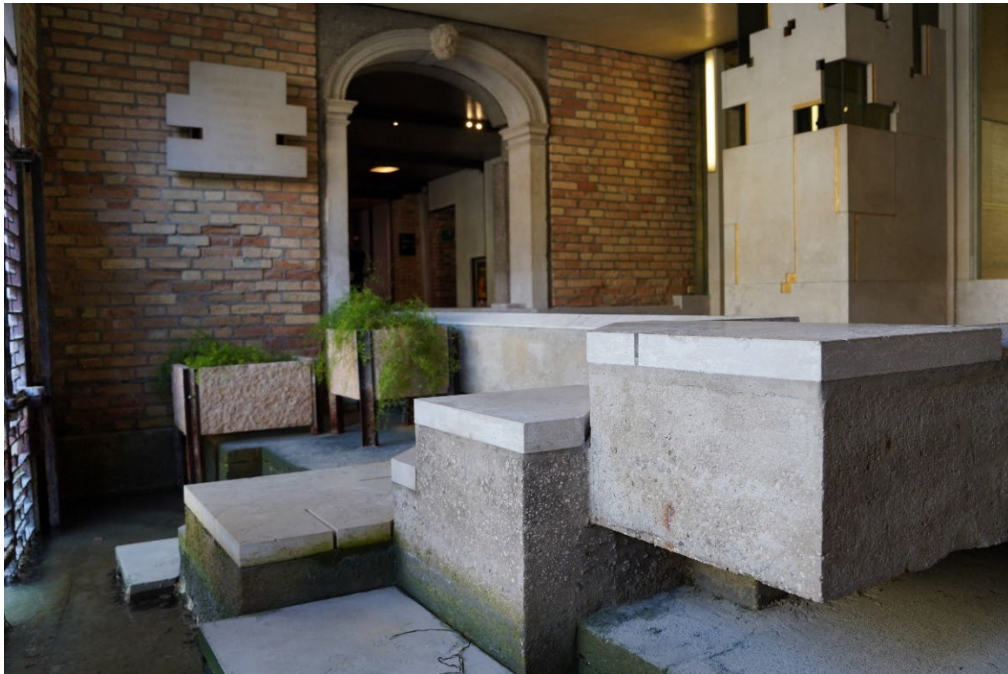
Fig. 23. The continued erosion of concrete reveals varying levels of texture and color, Querini Stampalia, Venice, Italy, 1963.
