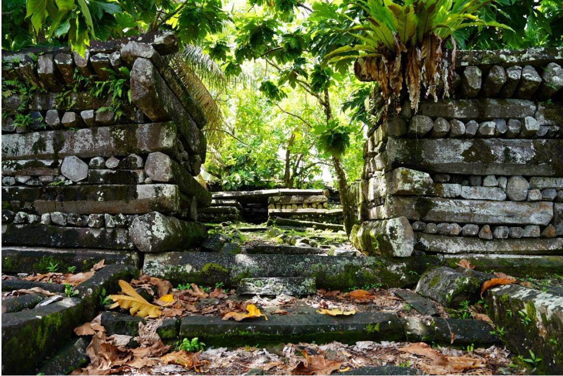
Fig. 43. The main entrance to the central courtyard remains standing, Nan Madol, Pohnpei, Micronesia, 1180.
