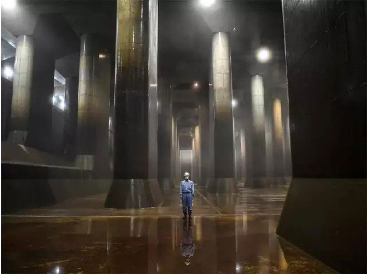
Fig. 28. The towering columns of the flood basin form a monumental hypostyle hall, G Cans, Kasukabe, Japan, 2006. 11
