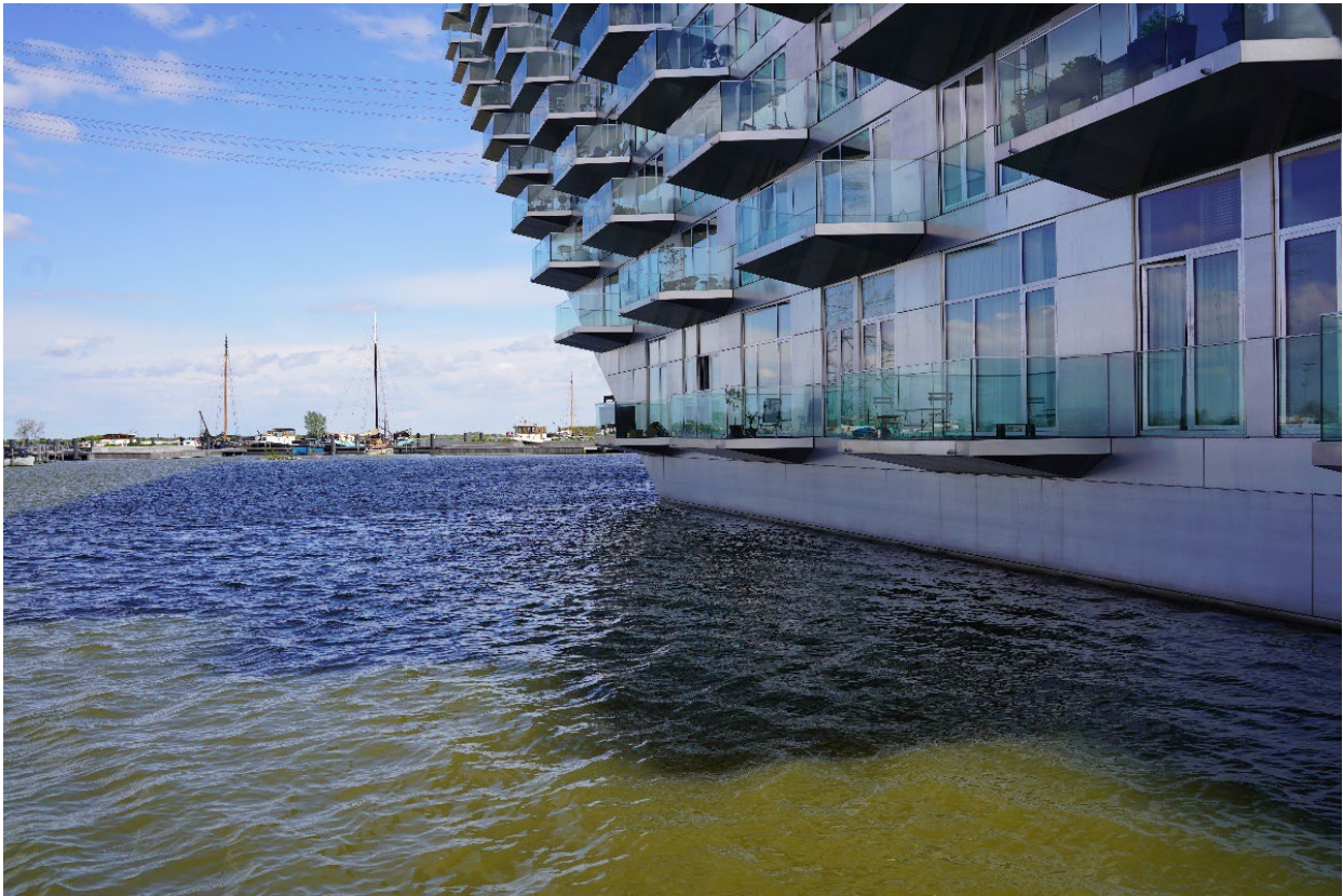
Fig. 8. The residence building rests in the water like a ship at dock, no change in building façade, Sluishuis Residential Building, Amsterdam, the Netherlands, 2022.
