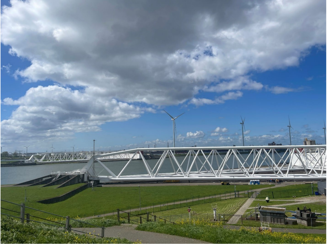
Fig. 3. View of the barrier resting on dry dock surrounded by rolling grass hills, Maeslant Barrier, Rotterdam, the Netherlands, 1997.
