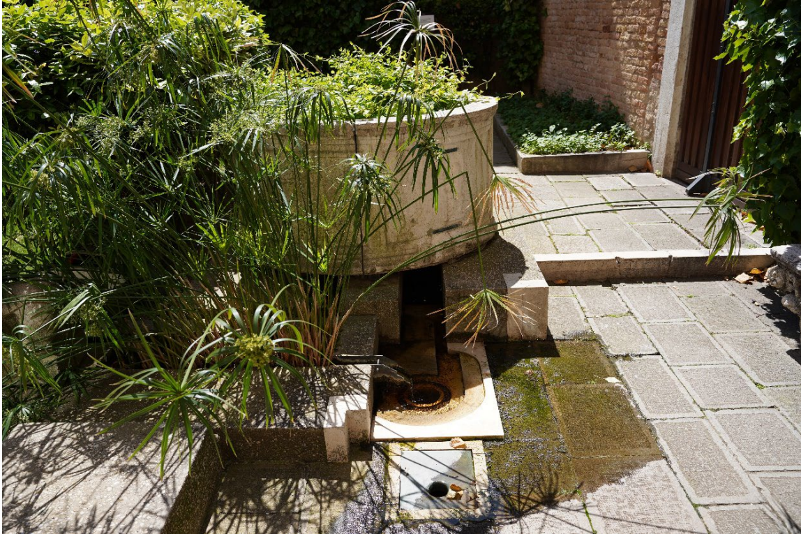
Fig. 25. At the end of the stone fountain sits a dry well and fountain drain where plants grow freely out of the seams, Querini Stampalia, Venice, Italy, 1963.
