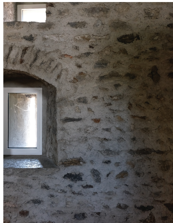
Previous Page: Inside the Museum's Permanent Exhibition Below (Left and Right): Rectangular Windows in Arched Openings
