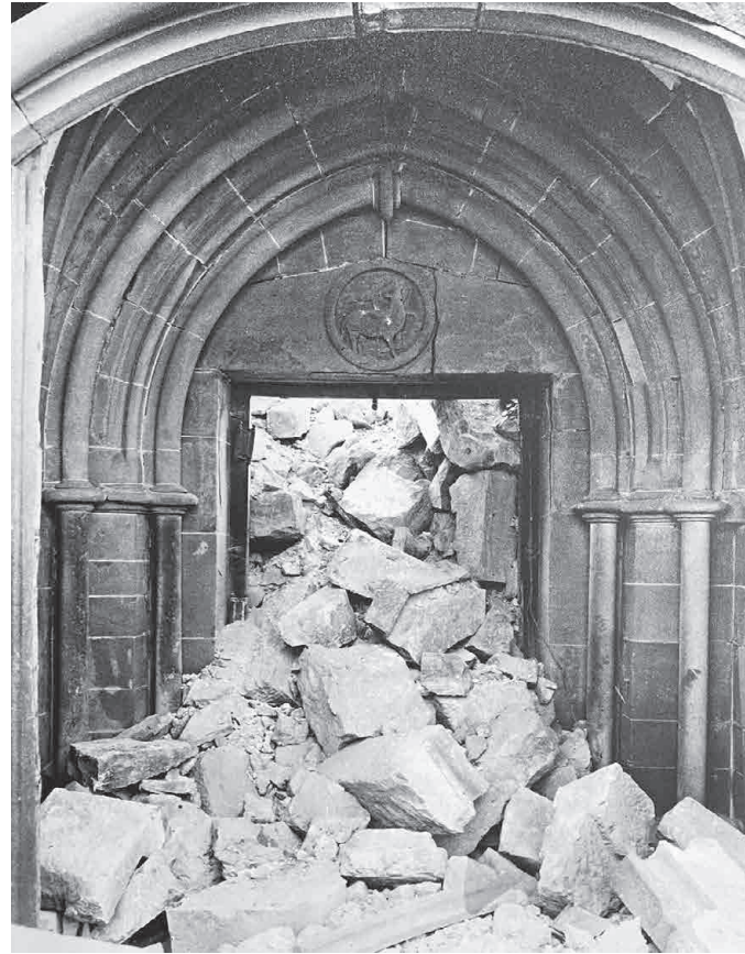
Right: South Portal with Rubble (Source: Annakirche Foundation in Düren)
