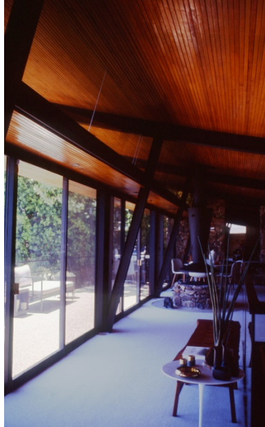
Fig. 6. Interior of Alexander House showcasing structural system and light shelf, Palm Springs, California. (photo: author)
