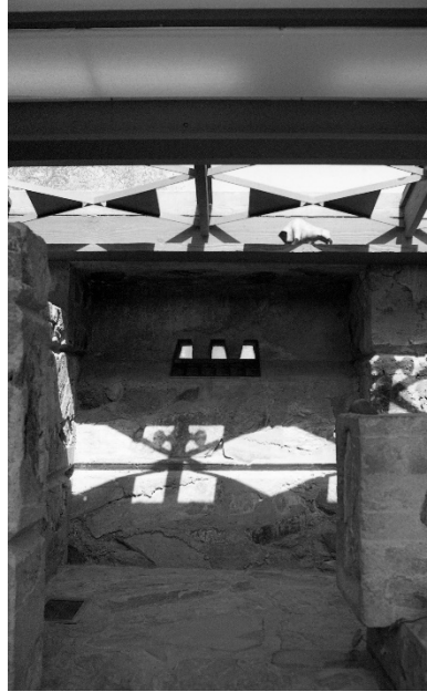
Fig. 6. Cast shadow from bracing members of the Garden Room at Taliesin West, Scottsdale, Arizona. (photo: author)
