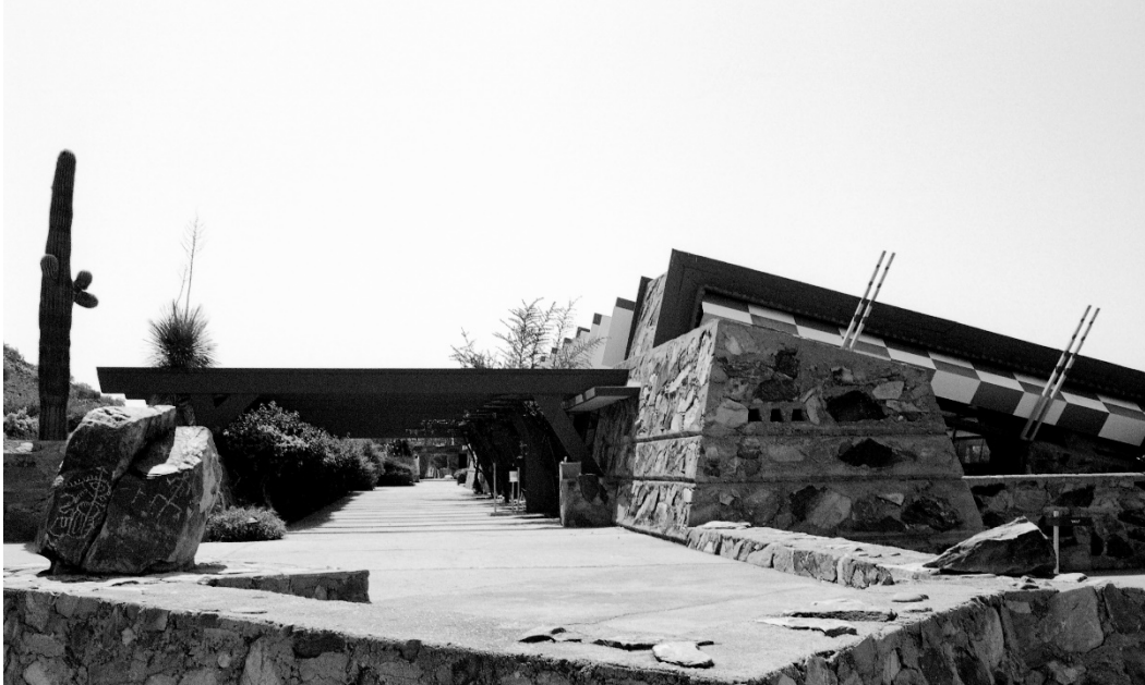
Fig. 2. Petroglyph atop prow to the right and Drafting Room at Taliesin West from the western elevation, Scottsdale, Arizona. (photo: author)
