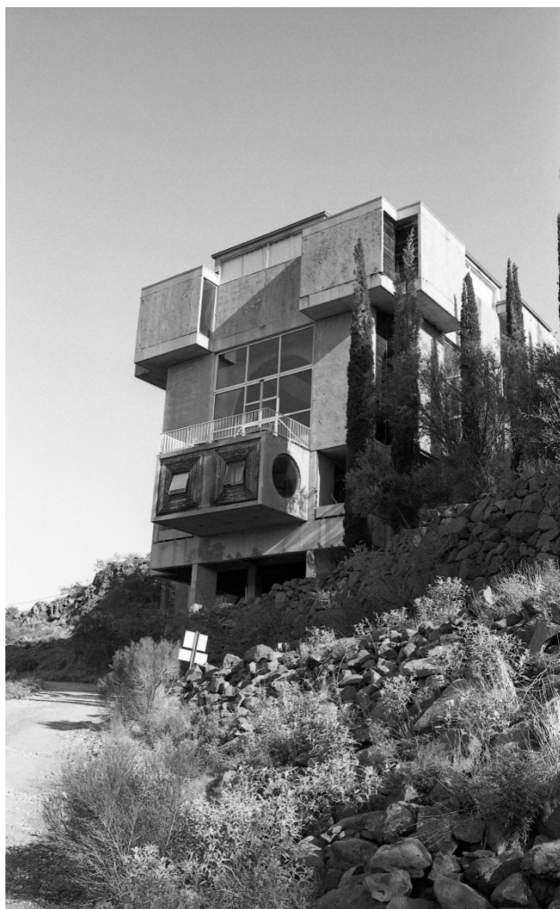
Fig. 7. Arcosanti main building and visitor's center, Yavapai County, Arizona. (photo: author)
