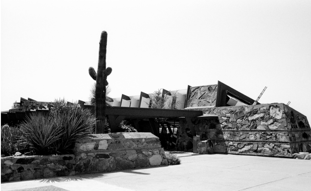
Fig. 10. Drafting Room from the southern and eastern elevation at Taliesin West, Scottsdale, Arizona. (photo: author)
