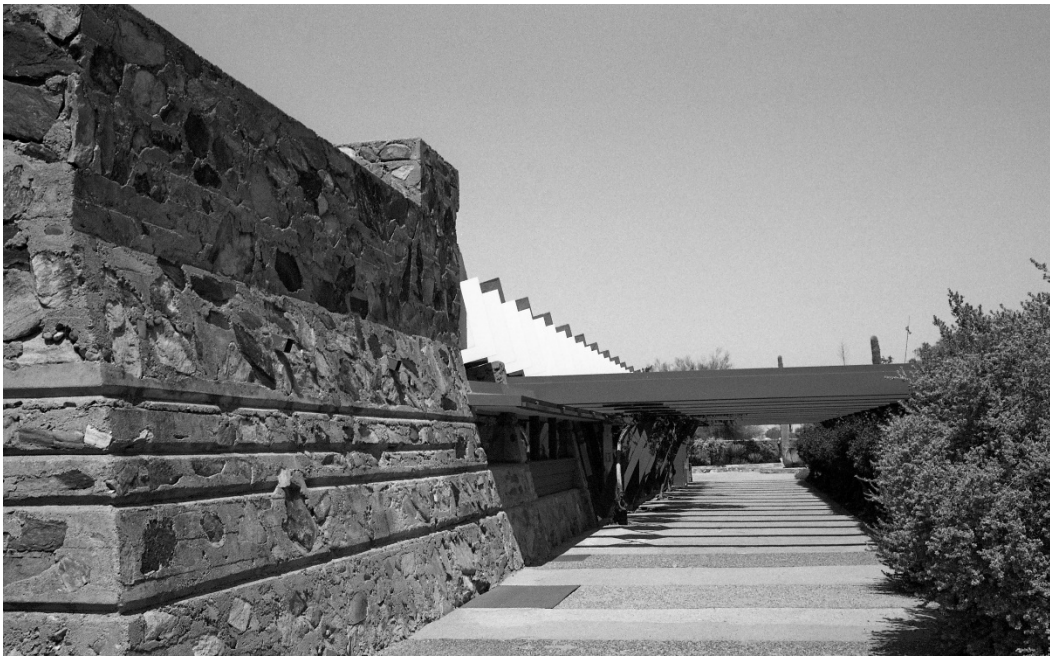
Fig. 4. Drafting Room at Taliesin West from the southern elevation with horizontal channels and pergola, Scottsdale, Arizona. (photo: author)
