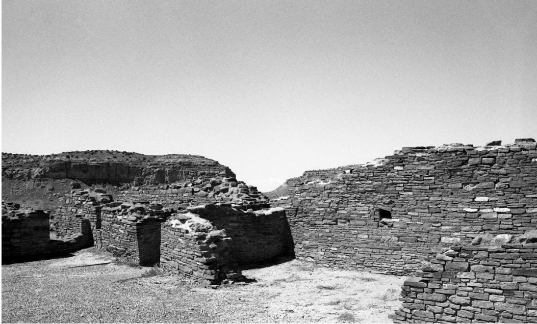
Fig. 10. Canyon wall opening framed by remaining masonry elements of Pueblo Bonito site, Nageezi, New Mexico. (photo: author)
