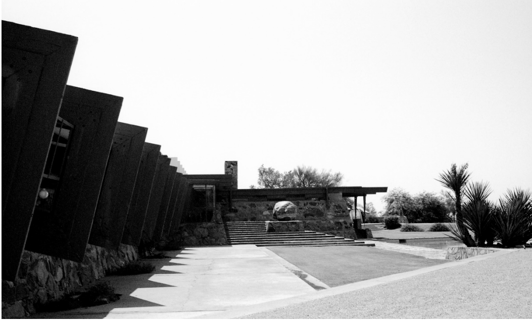
Fig. 8. Mainframe rafters of Drafting Room from northern elevation at Taliesin West, Scottsdale, Arizona. (photo: author)
