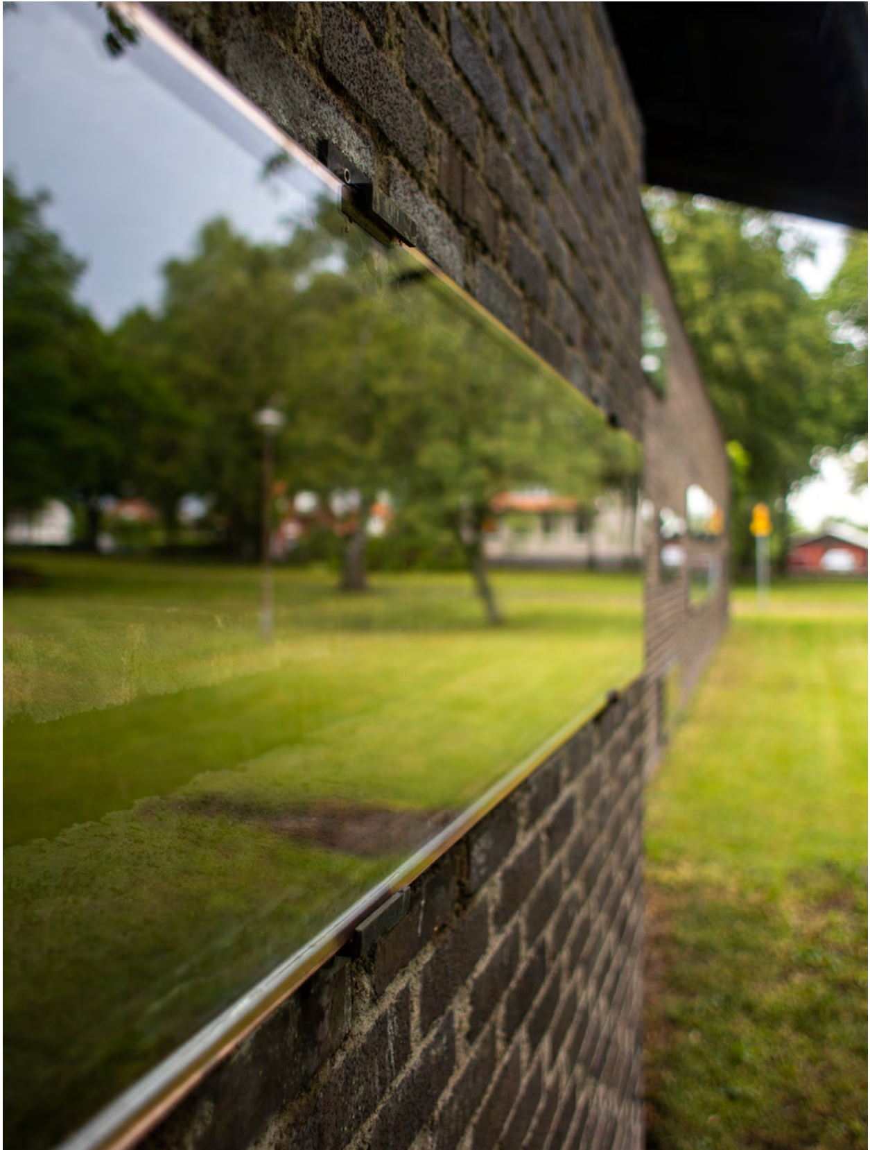
Fig. 17 Sigurd Lewerentz, exterior windows along the offices, Saint Peter, Klippan, 1966. Photograph by author, 2019.
