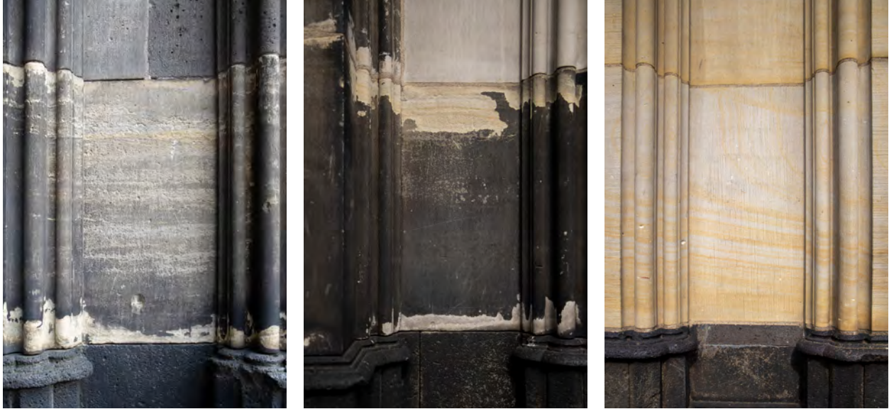
Fig. 24-26 Original, transitional, replaced stone, Cologne Cathedral, Cologne, 1880. Photograph by author, 2019.
