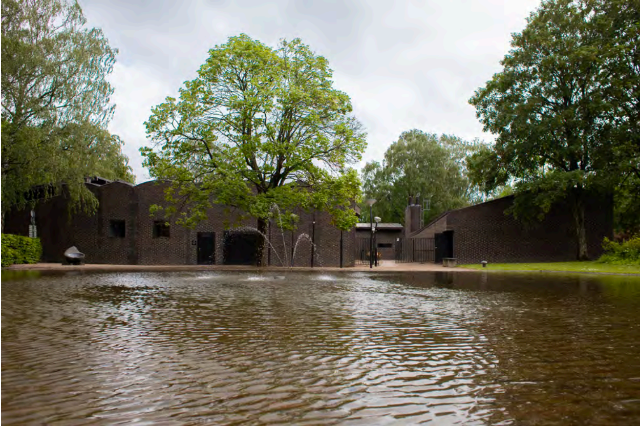
Fig. 04 Sigurd Lewerentz, western facade, Saint Peter, Klippan, 1966. Photograph by author, 2019.
