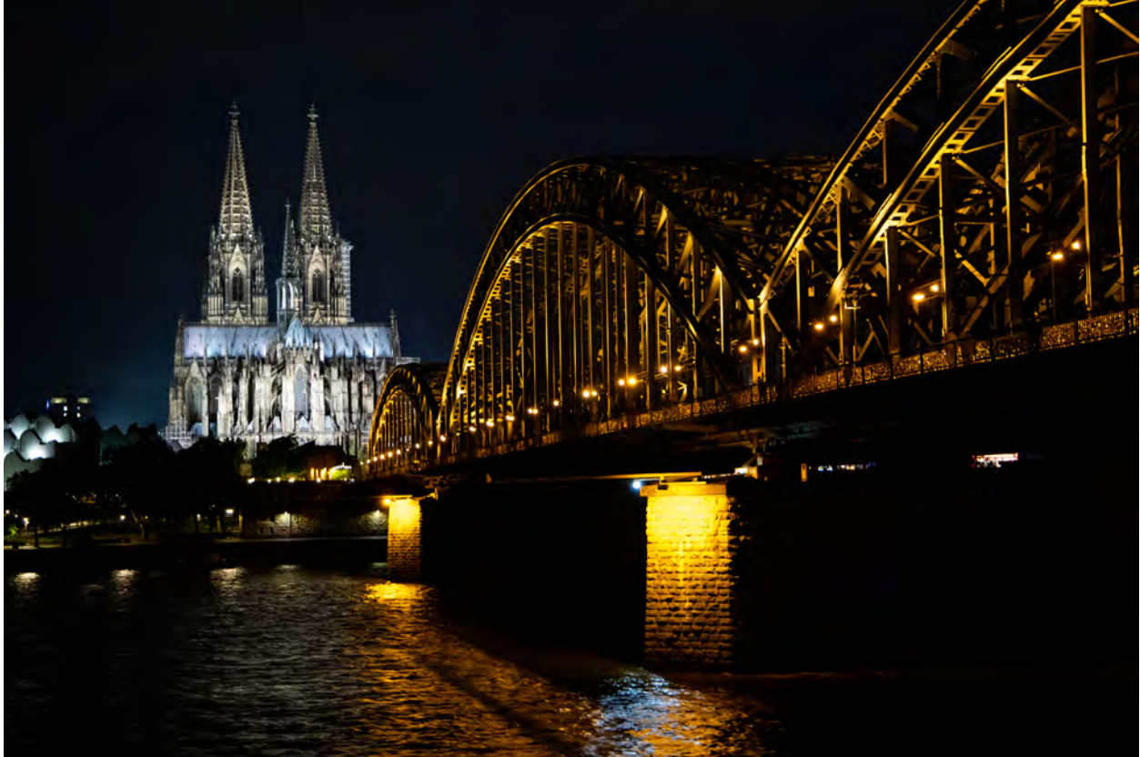
Fig. 18 Night view along Hohenzollern Bridge, Cologne Cathedral, Cologne, 1880. Photograph by author, 2019.
