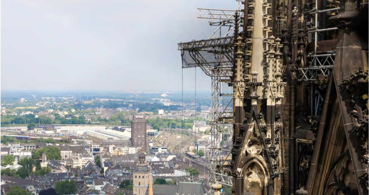
Fig. 29 Scaffolding on the north tower, Cologne Cathedral, Cologne, 1880. Photograph by author, 2019.
