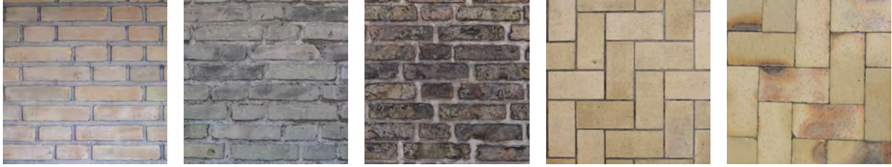
Fig. 22-26 P.V. Jensen-Klint, material palette, Grundtvig's Church, Copenhagen, 1940. From left: interior, exterior, neighboring structures, interior floor, exterior paving Photographs by author, 2019.
