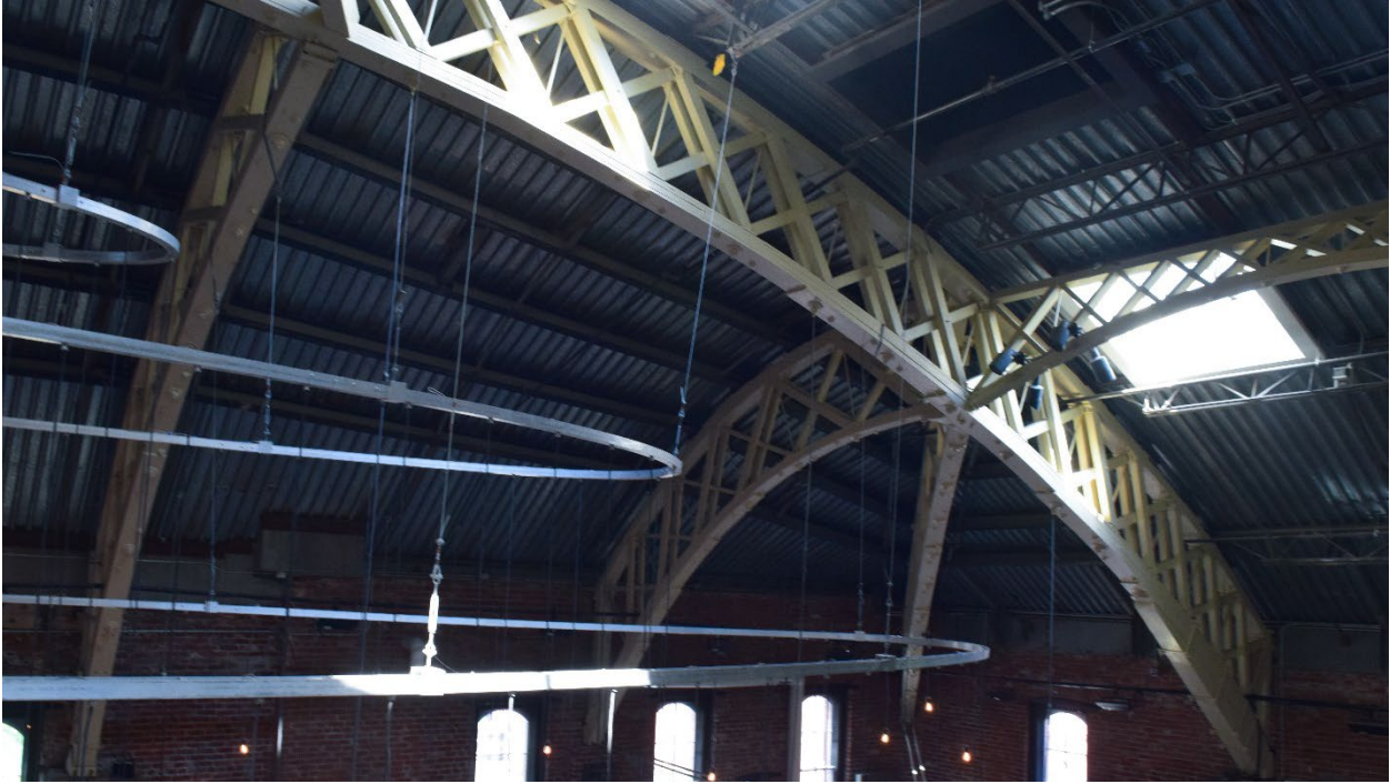
Fig. 5, Martin & McCaw, Interior showing wooden truss system, The Armory Annex, Portland, OR, 1891.
