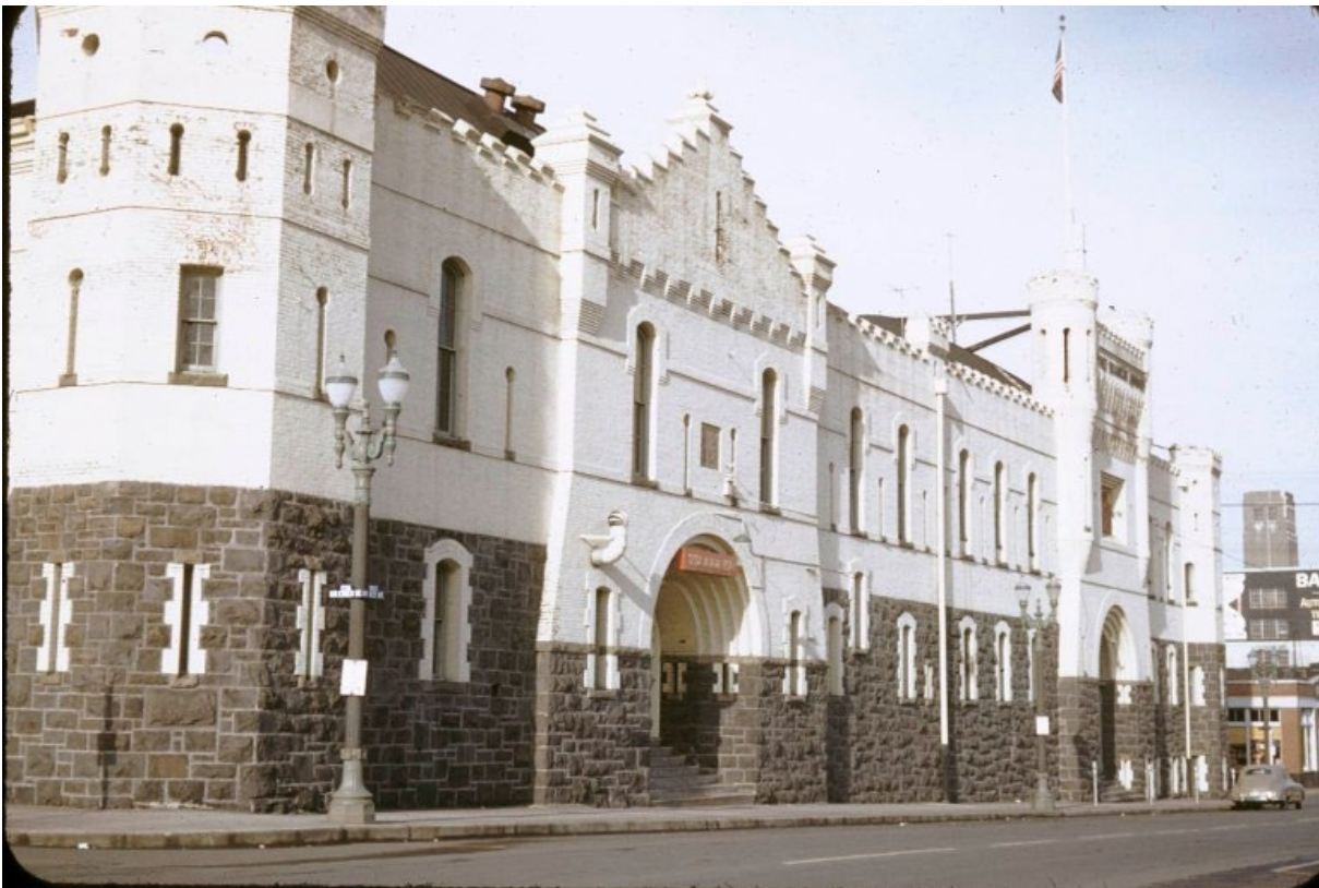
Fig. 3, Martin & McCaw, The Armory Annex Whitewashed, The Armory Annex, Portland, OR, 1891. Source: https://vintageportland.wordpress.com/2012/10/15/oregon-national-guard-armory-1953/
