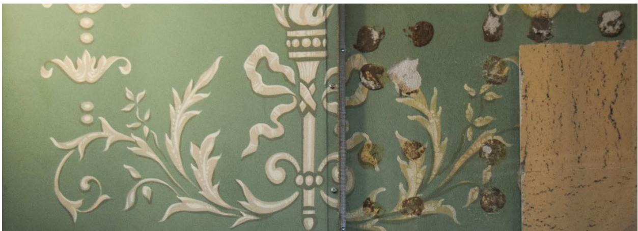
Fig. 11-15, interior of House and Seante Chamber after Renovation, Elijah Meyers, Colorado State Capitol Building, Denver, CO, 1894.
