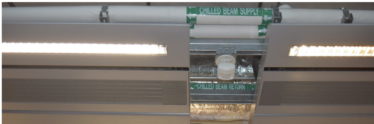
Fig. 10, Martin & McCaw, interior showing chilled beam supply, the Armory Annex, Portland, OR, 1891.
