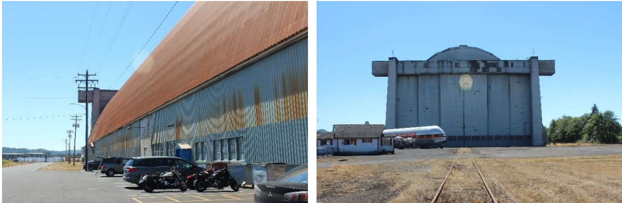
Fig. 2. Exterior views of the hangar, disrepair visible, Tillamook, OR, 2021.
