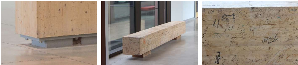
Fig. 19. Leers Weinzapfel Associates, bottom of glulam column in the Commons, John W. Olver Design Building, Amherst, MA, 2021.
