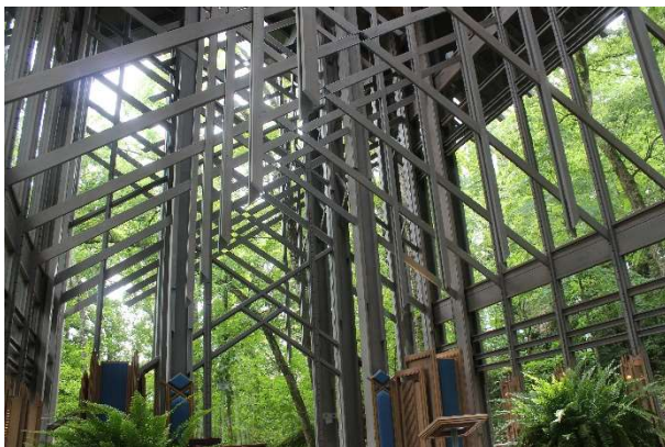
Fig. 5. E. Fay Jones, view of the cross bracing from a seated position in the pews, Thorncrown Chapel, Eureka Springs, AR, 2021.
