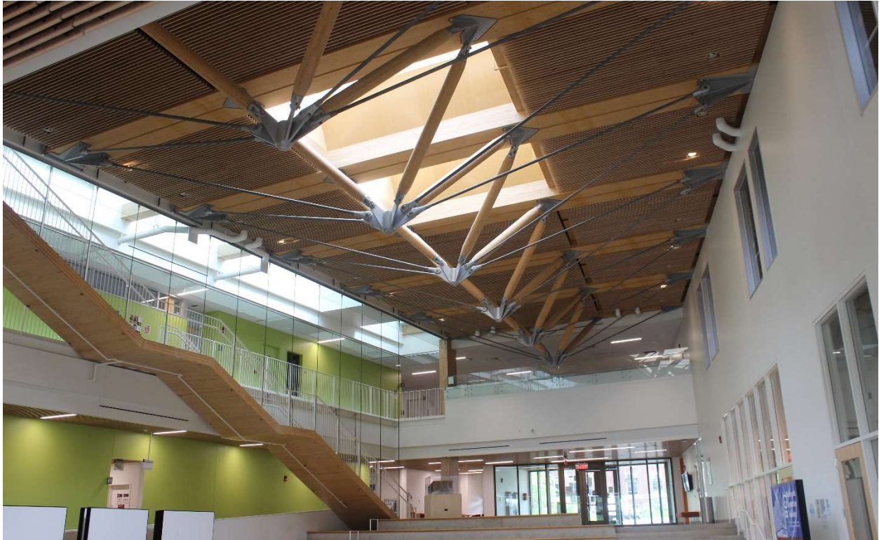
Fig. 4. Leers Weinzapfel Associates, picture of the Commons looking up towards the zipper truss supporting the ceiling, John W. Olver Design Building, Amherst, MA, 2021.
