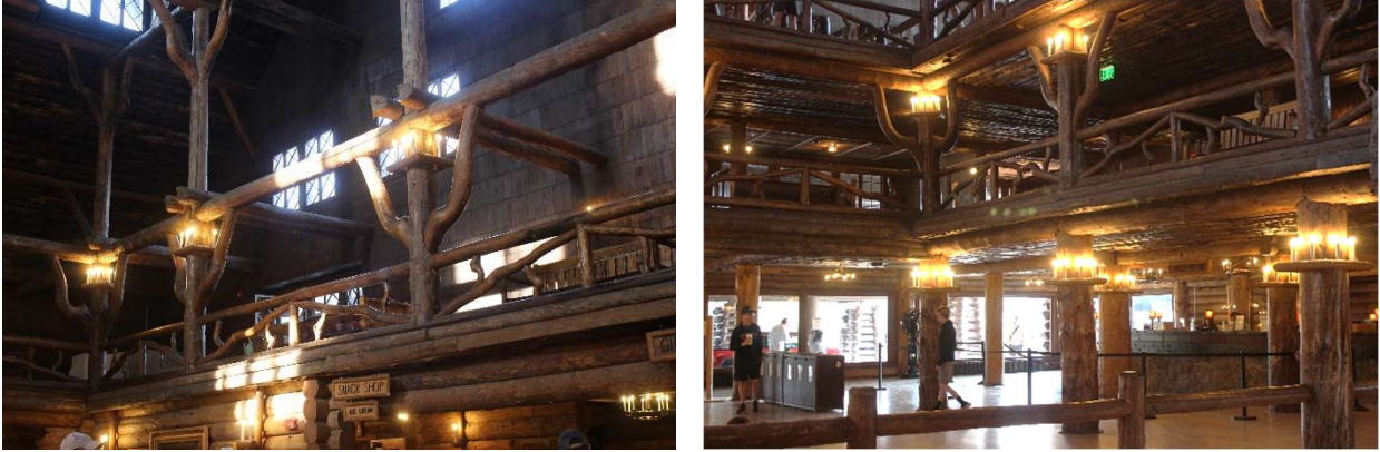
Fig. 8-9. Robert C. Reamer, images of the knotty wood bracing and the lobby columns, Old Faithful Inn, Yellowstone National Park, WY, 2021.
