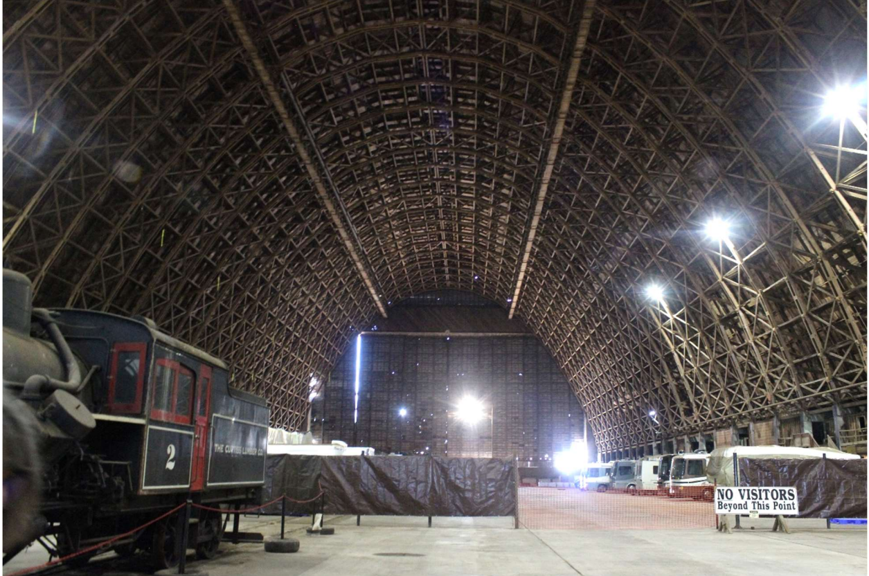
Fig. 3. Southwest view from inside the hangar, Tillamook, OR, 2021.
