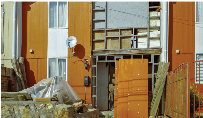
Fig. 12. ELEMENTAL, Villa Verde, Constitución, Chile, 2010. One of the units under construction, the exterior façade removed exposing the timber frame.
