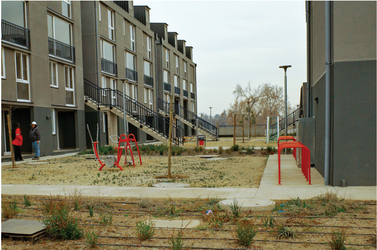
Fig. 14. ELEMENTAL, Los Presidentes, Santiago, Chile, 2025. Two days after construction. The courtyard is car-free being replaced by bike racks and outdoor exercise equipment.
