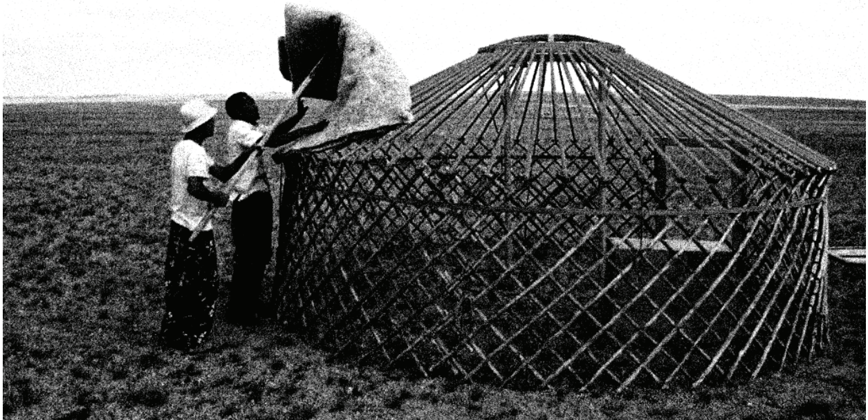
Fig. 11. Mongolian countryside. Two men begin applying layers of felt to the structure. Original photo by Travel Buddies Mongolia, 2023.
