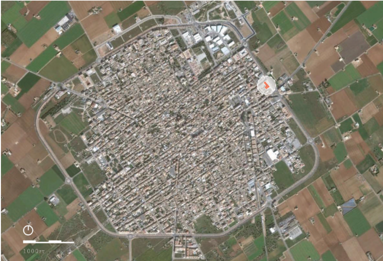
Fig. 2. RIPOLLTIZON Architects, aerial view of project in context, Social Housing in Sa Pobla, Mallorca, Spain, 2012.
