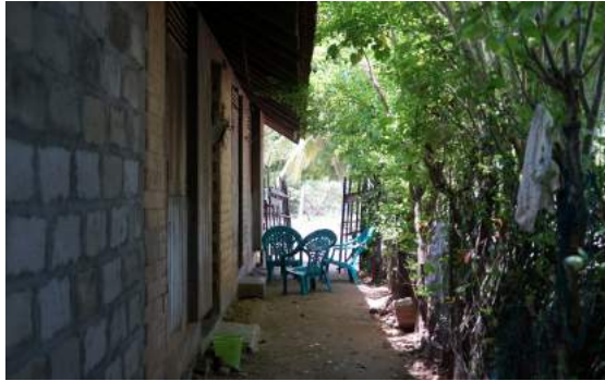
Fig. 22. Shigeru Ban, seating area in a side yard, Post-Tsunami Housing, Kirinda, Sri Lanka, 2007.
