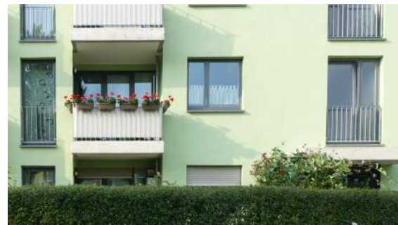
Fig. 19. ASTOC Architects and Planners, windows and balconies and balconettes, Cologne, Germany, 2012.
