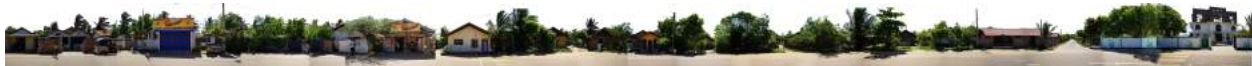
Fig. 7. Shigeru Ban, elevations along main road looking northwest, Post-Tsunami Housing, Kirinda, Sri Lanka, 2008.
