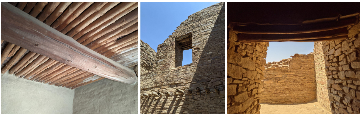
Fig. 7. Ancestral Puebloans, (photographs: Tunnell) reconstructed interior, original timber structural elements, pine doorway header , Pueblo Bonito, Chaco Canyon, NM, 850-1150.
