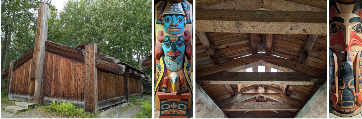
Fig. 8. Eyak, Haida, Tsimshian, & Tlingit, (photographs: Tunnell) cedar plank house with carved columns & heavy timber structure , Alaska Native Heritage Center, Anchorage, AK, 700-1800.
