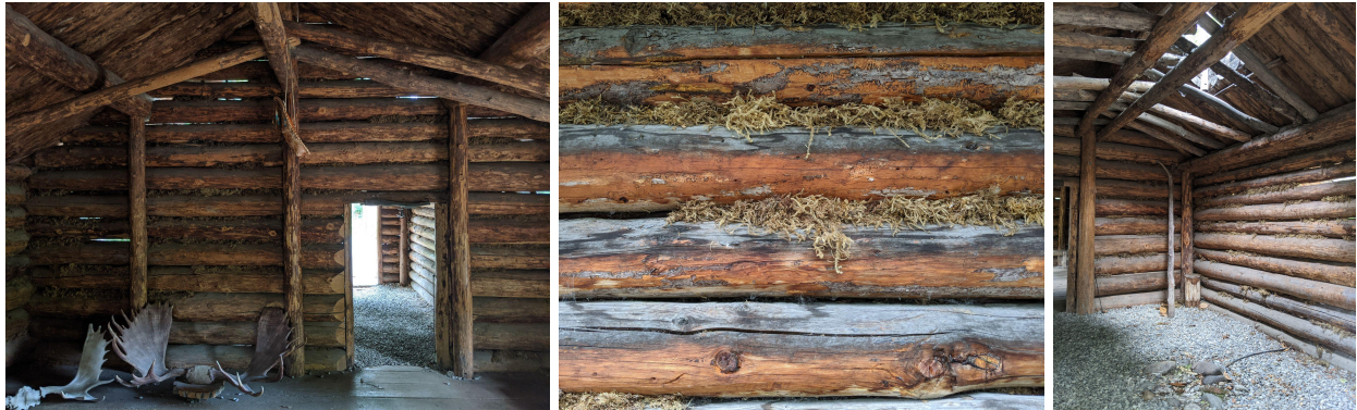
Fig. 5. Athabascan, (photographs: Tunnell) timber structure, moss filling, & fire ventilation, Athabascan winter home, Alaska Native Heritage Center, Anchorage, AK, 700-1800.
