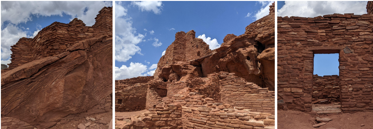
Fig. 8. Ancestral Puebloans, (photographs: Tunnell) Moenkopi sandstone masonry & door frame details, Wupatki Pueblo, Flagstaff, AZ, 1106-1225.
