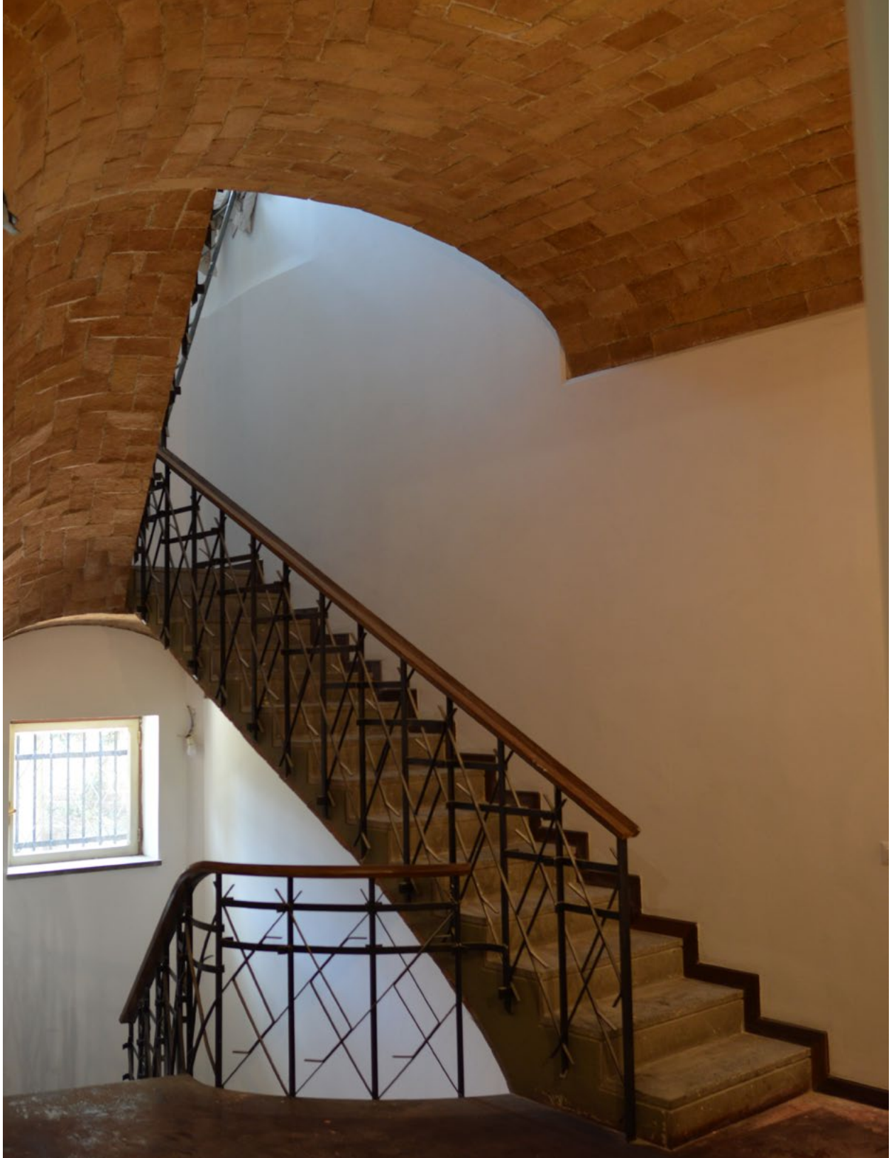
Fig. 6. Paolo Portoghesi, stair with herringbone brick vaults, Casa Baldi, Rome, Italy, 1959
