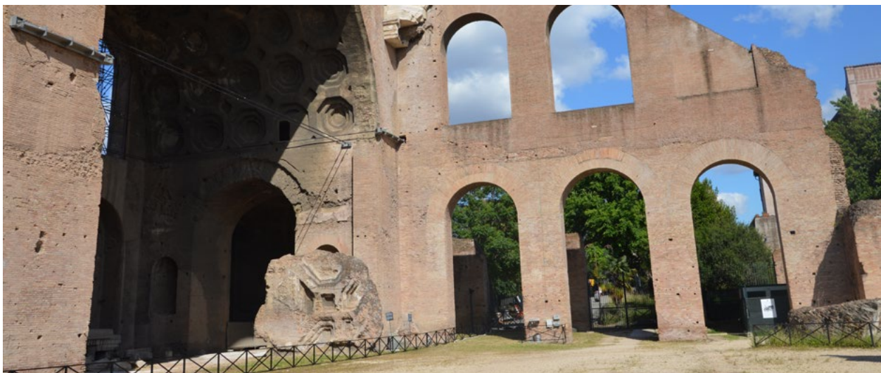
Fig. 1. (top) Roman Colisseum showing radial vaults, (middle) Roman Pantheon, intradose of the dome and oculus, (bottom) Basilica of Constantine, barrel vault and end wall
