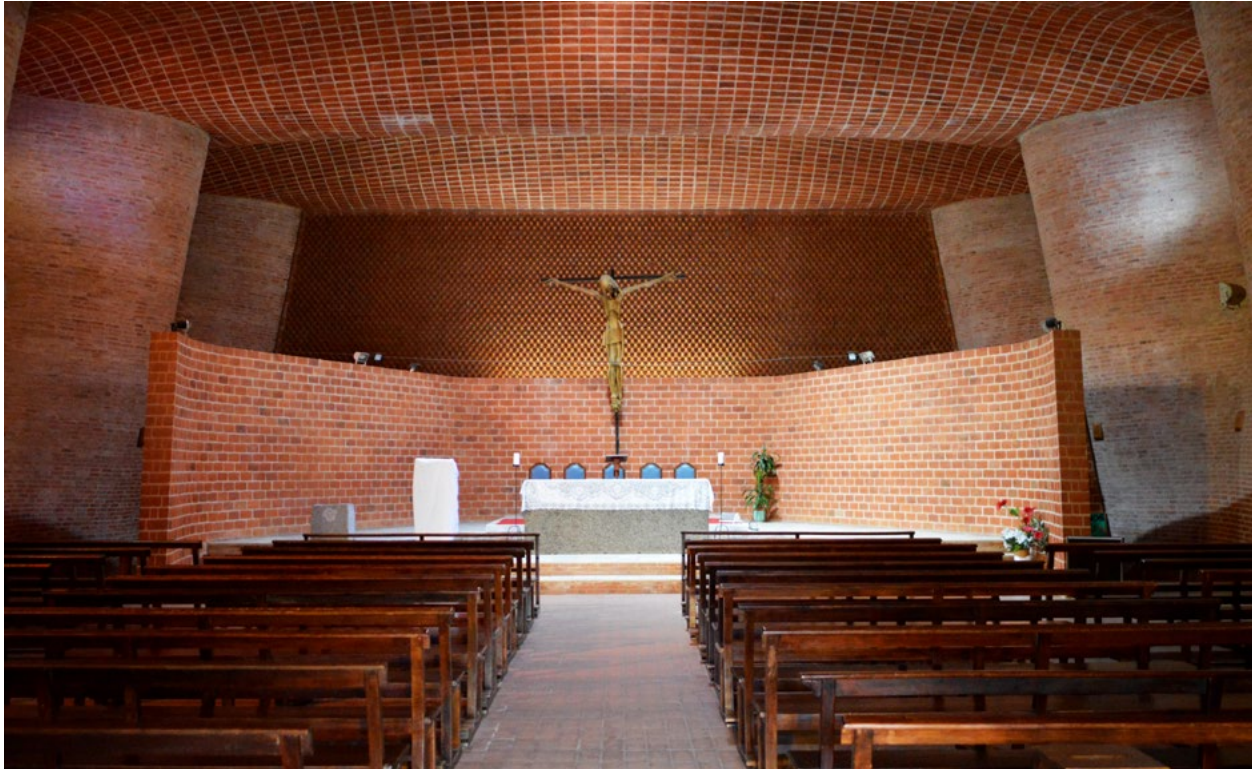
Fig. 9. Eladio Dieste, view down the nave to the chancel showing canted brick, Church of Cristo Obrero, Atlantida, Uruguay, 1958
