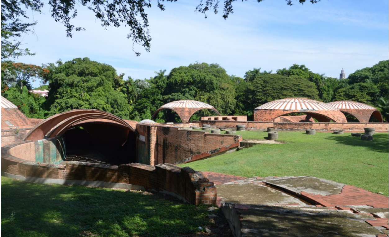
Fig. 3. Vittorio Garatti, entrance with domed pods beyond, School of Ballet, Havana, Cuba, 1961
