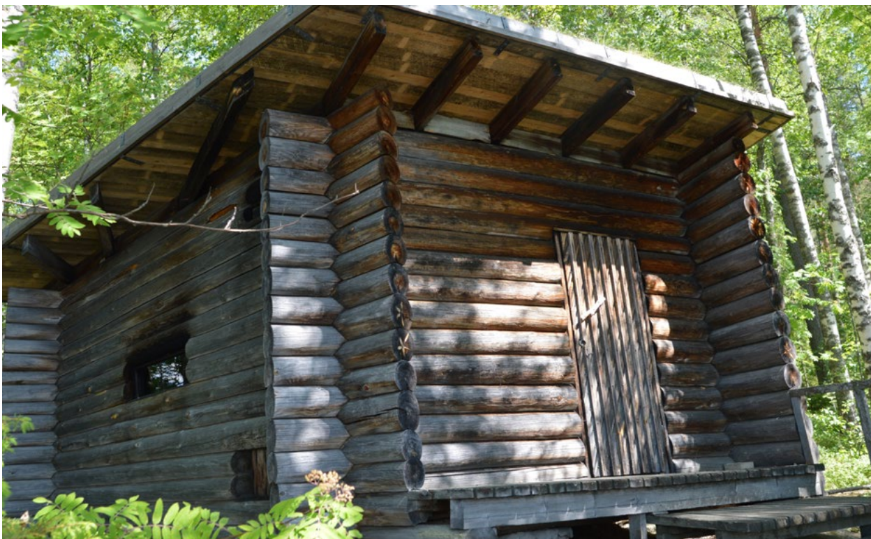
Fig. 3. log construction of the sauna, Muuratsalo, Finland
