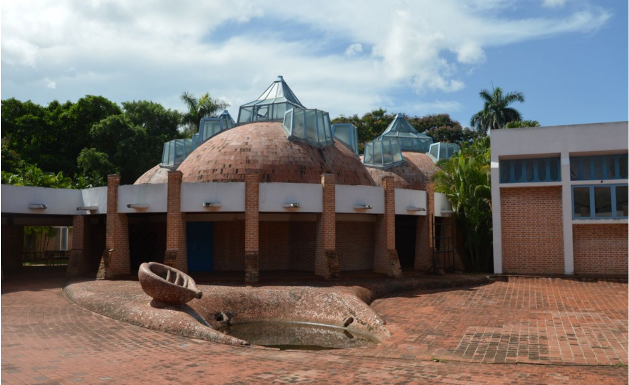
Fig. 10. Ricardo Porro, papaya shaped fountain with brick-domed studio beyond, School of Plastic Arts, Havana, Cuba, 1961
