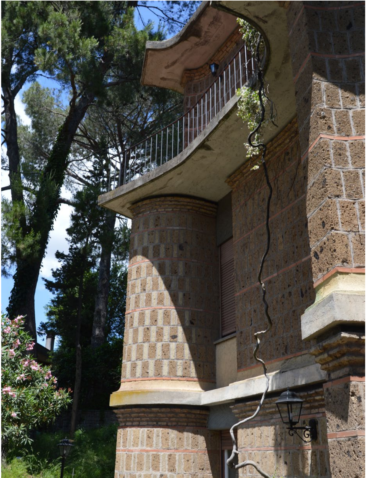
Fig. 3. Paolo Portoghesi, wall detail showing tufa stone patterns, Casa Baldi, Rome, Italy, 1959
