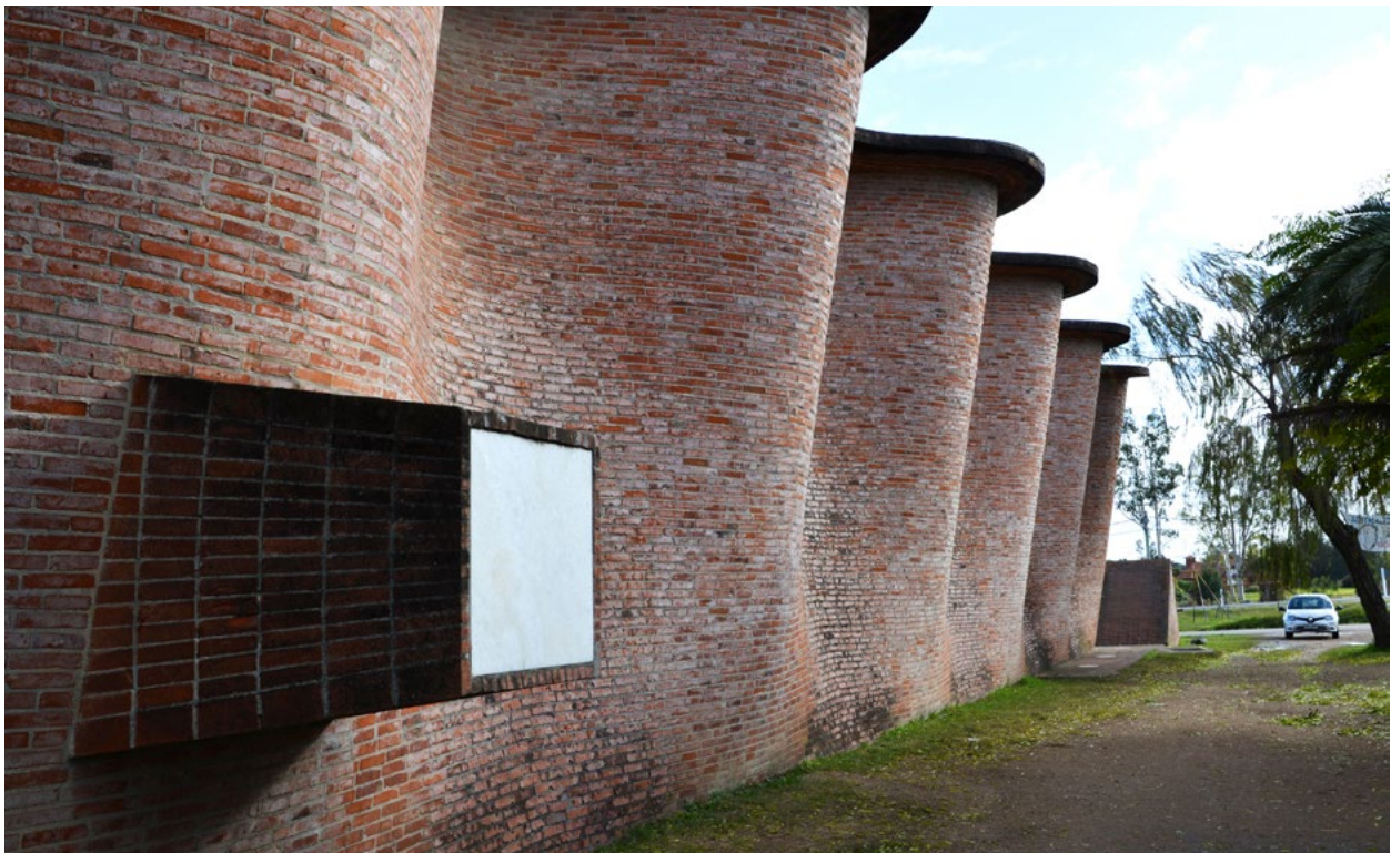
Fig. 5. Eladio Dieste, left side wall light box for the Virgin Mary figure, Church of Cristo Obrero, Atlantida, Uruguay, 1958
