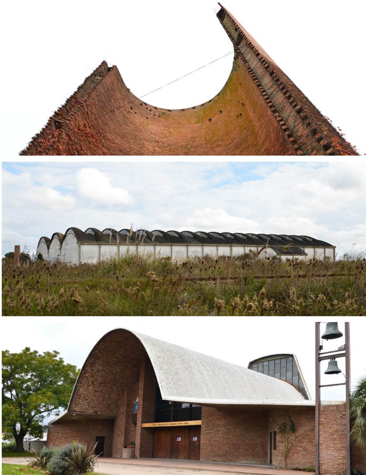
Fig. 1. Eladio Dieste, (top) unfinished church apse, (middle) Gaussian vaults at wool factory in the countryside, (bottom) freestanding vault at Montevideo church, date unknown
