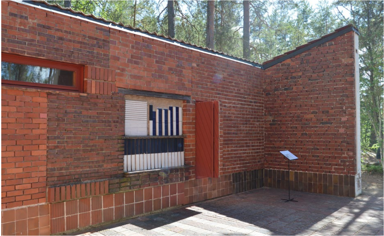
Fig. 13. Alvar Aalto, brick and tile patterning at the bedroom wing, Experimental House, Muuratsalo, Finland, 1952
