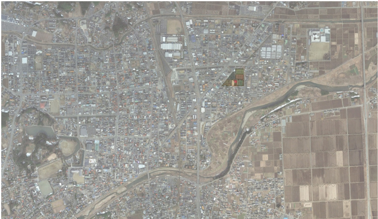
Fig. 6. Klein Dytham Architects, siting within the town of Soma around one of the few green spaces in the community, Soma Home for All, Soma, Japan, 2016.
