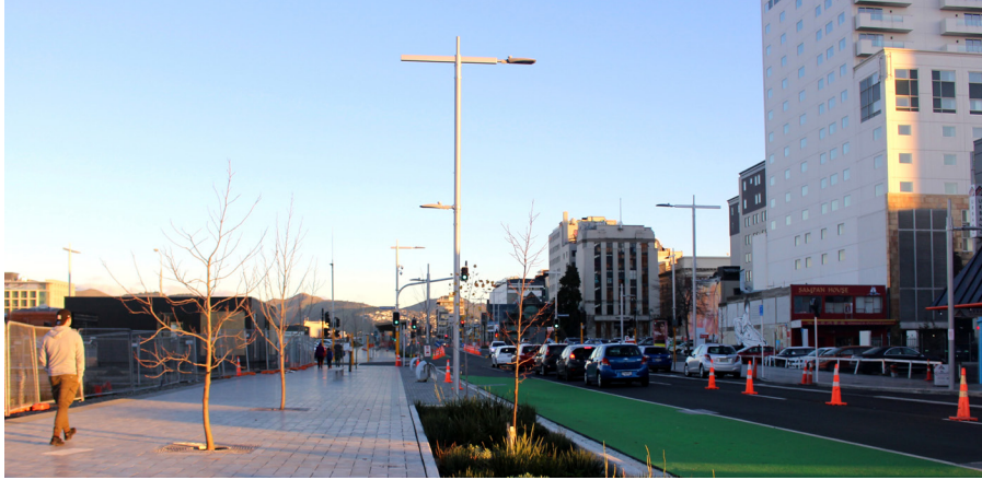
Fig. 7. infrastructure 'complete street' renovation underway, Christchurch, New Zealand.
