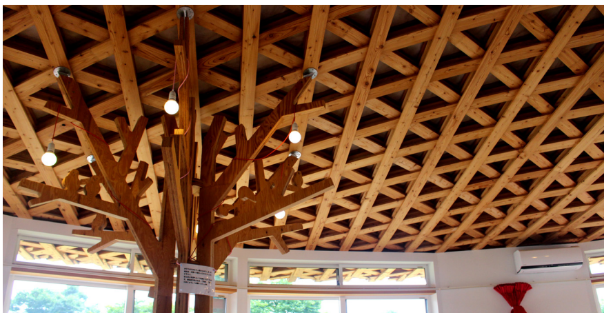
Fig. 5. Klein Dytham Architects, columns disguised as trees, Soma Home for All, Soma, Japan, 2016.
