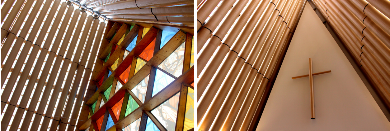
Fig. 16. Shigeru Ban, front and back walls of the Cathedral framed by cardboard tube beams, Transitional Cathedral, Christchurch, New Zealand, 2013.
