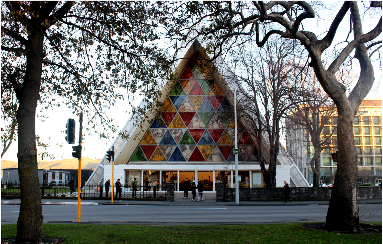
Fig. 1. Shigeru Ban, front elevation, Transitional Cathedral, Christchurch, New Zealand, 2013.
