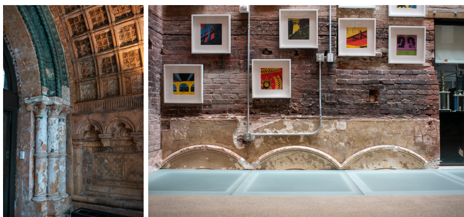
Fig. 9. KoningEizenberg Architects, details of existing revealed stonework, Pittsburgh, PA, 2019.
