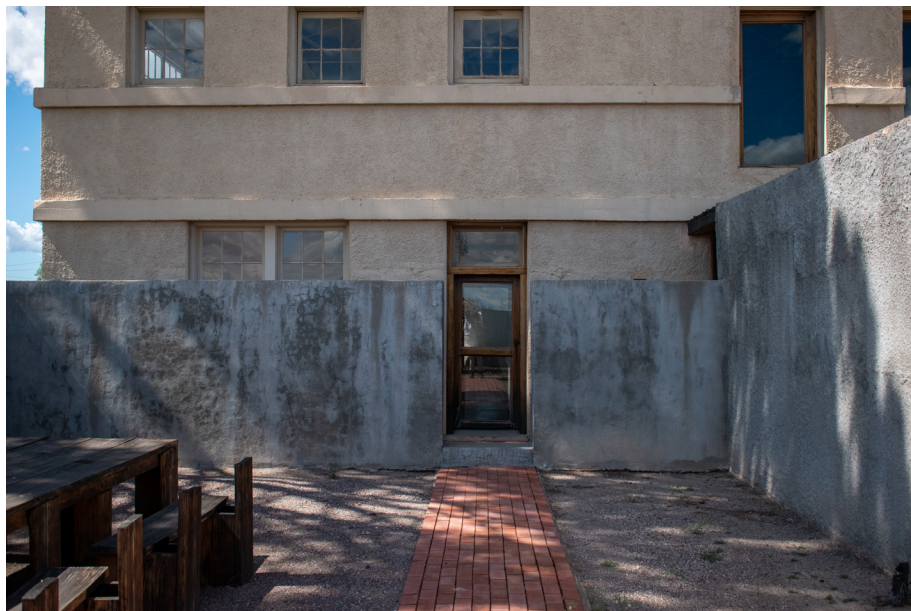
Fig. 9. Donald Judd, view from courtyard toward the Arena's rear entrance, The Chinati Foundation, Marfa, TX, 1930s-1980s.
