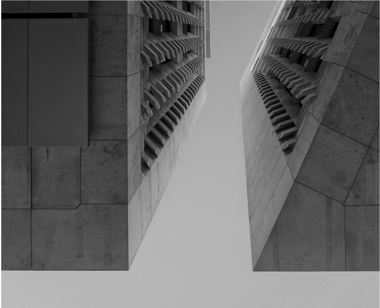
Fig. 1. Renzo Piano Building Workshop, La Valletta City Gate, La Valletta, Malta, 2009 - 2015
