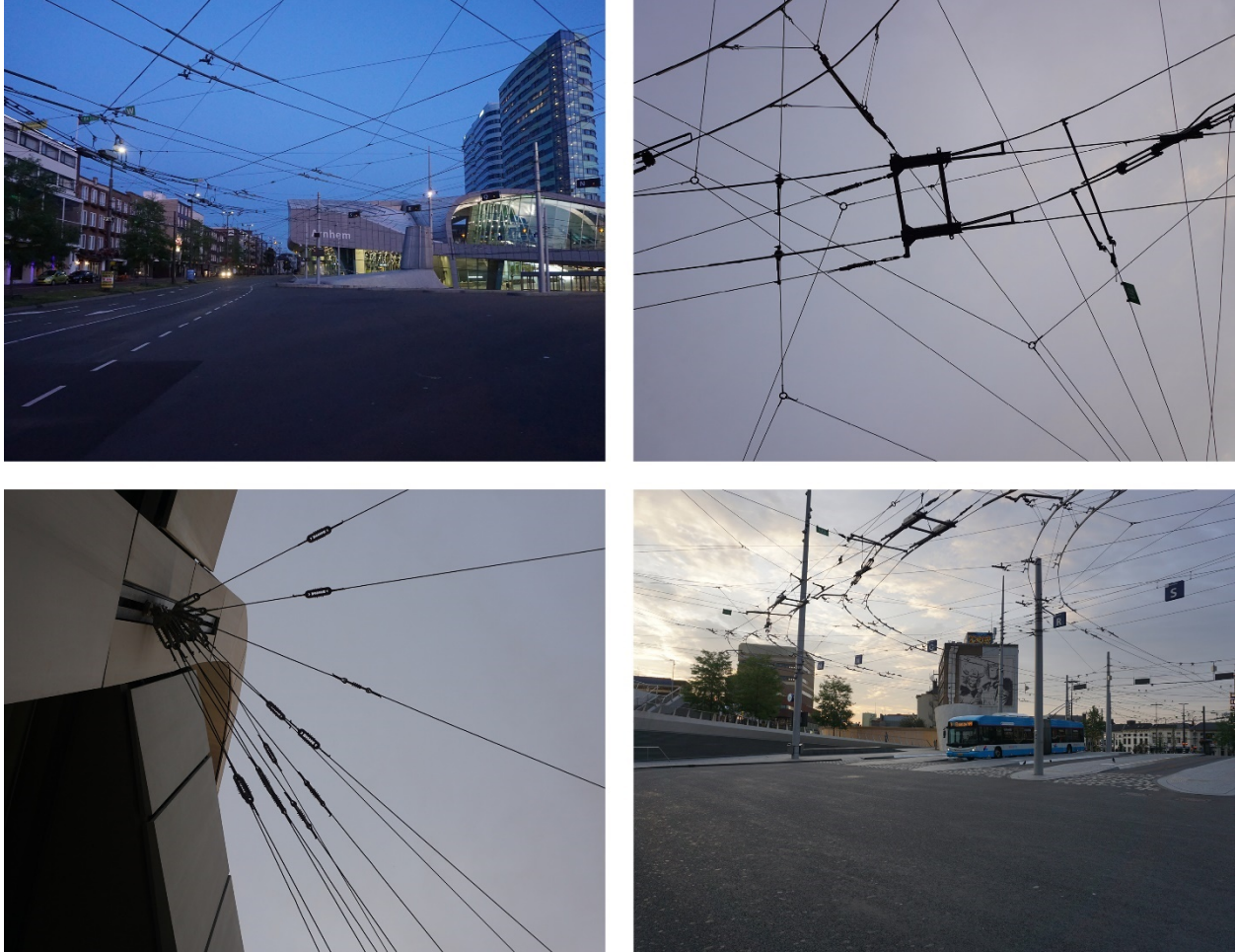
Fig. 19-22. UNStudio, Spiderweb Cable Lines, Arnhem Central Station, Arnhem, Netherlands, 1996 - 2015
