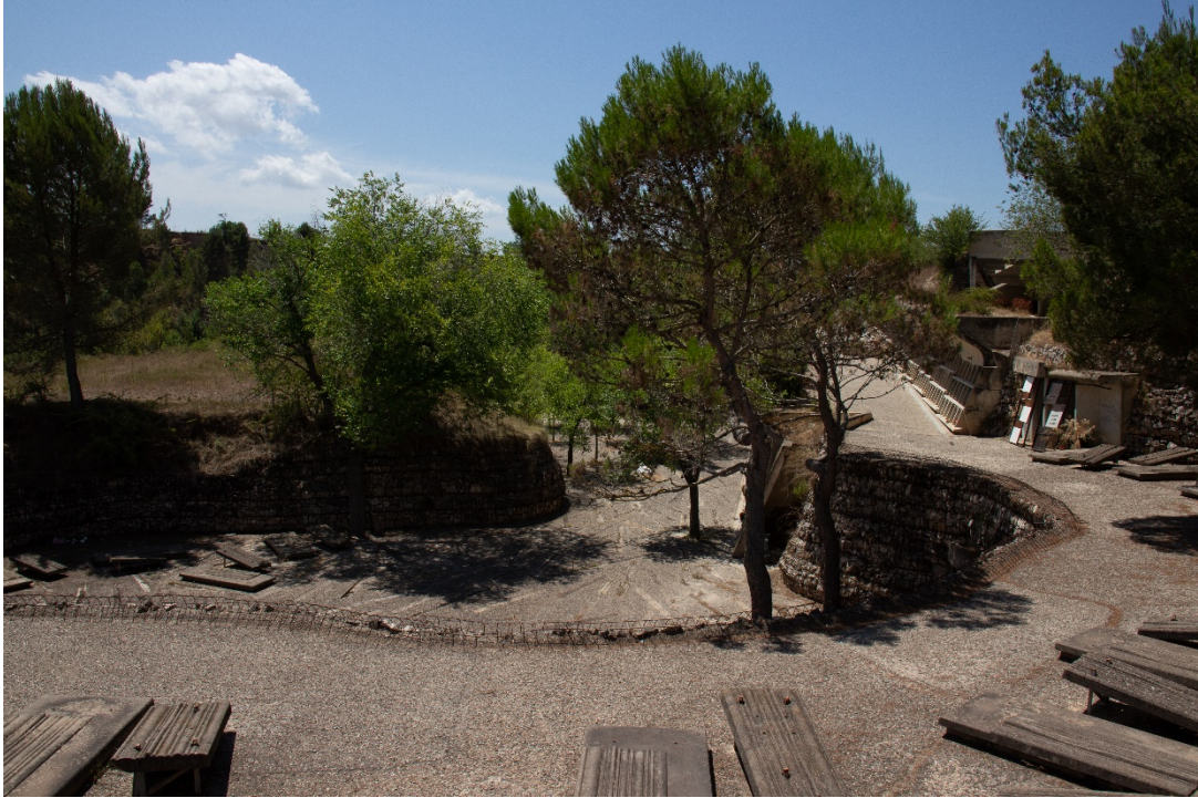
Fig. 11 - Terraces of concrete roofs
