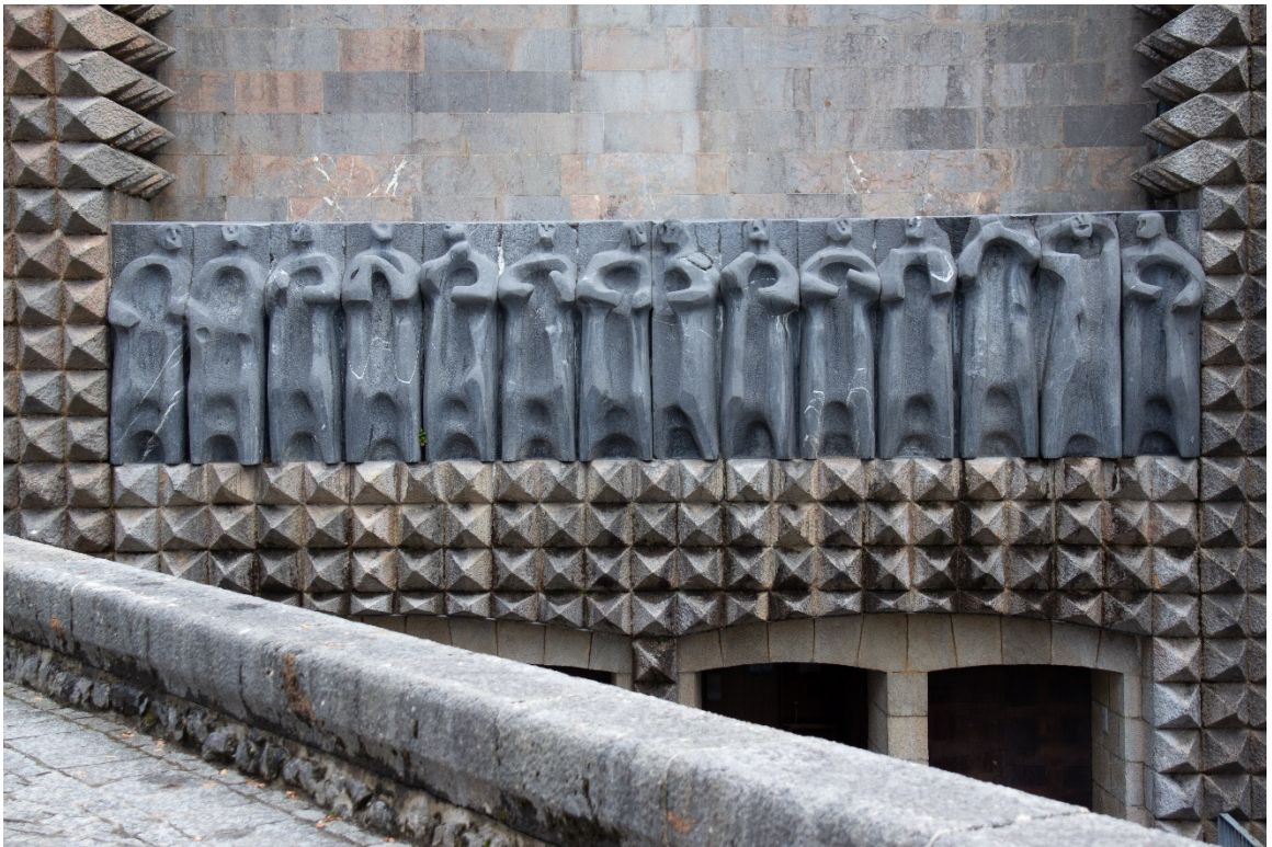
Fig. 35, 36 - Spikes at the sanctuary
