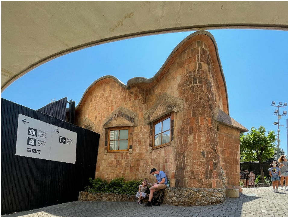
Fig 26 - Exterior of school building
