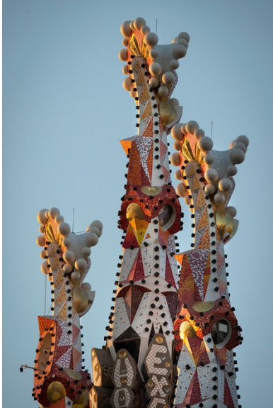
Fig. 9 - Close up of colored mosaic tiles on pinnacle of towers, Photo from Basilica de la Sagrada Familia organization
