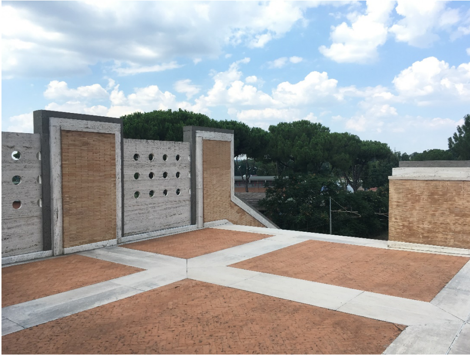
Fig. 27 - Typical long and thin Roman brick and travertine (white limestone)
