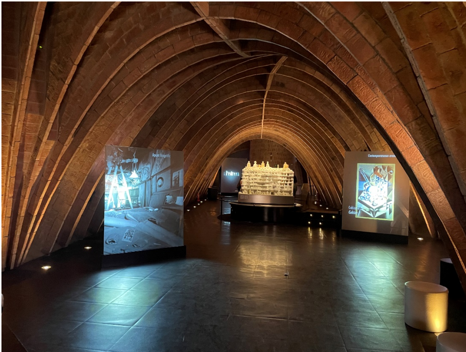
Fig. 19, 20, 21 - Ribbed vaults under Casa Mila's roof, attic is currently a museum.
