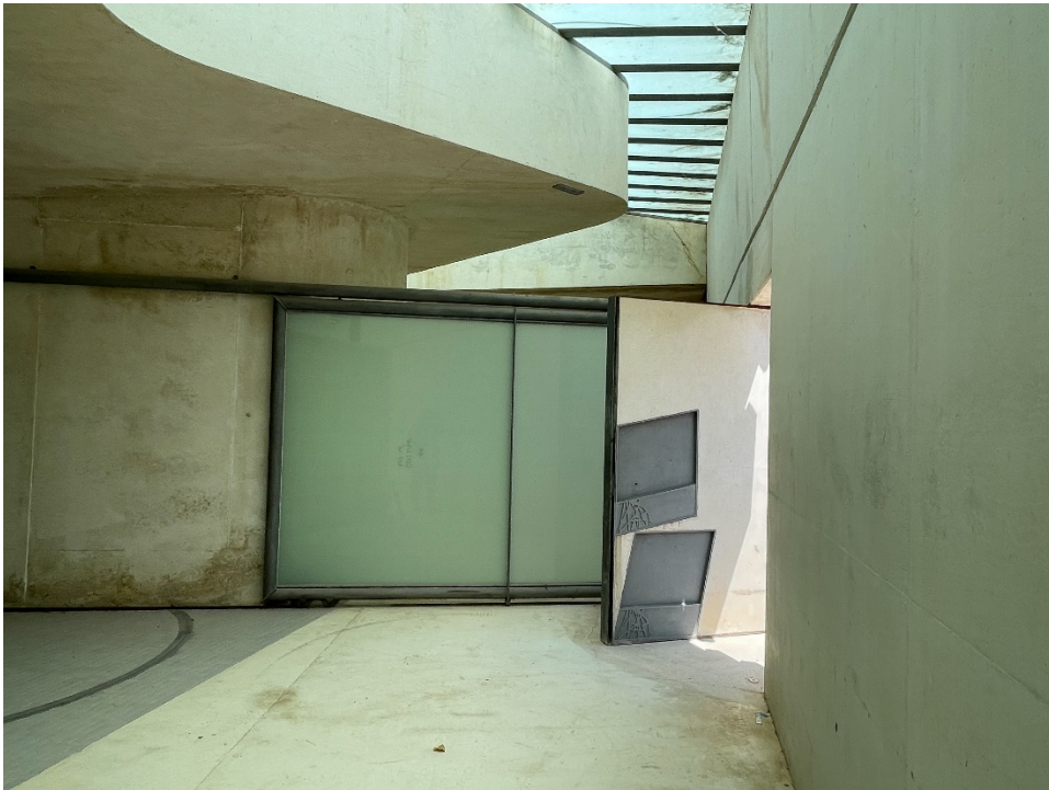
Fig. 7 - Interior of unfinished service building
