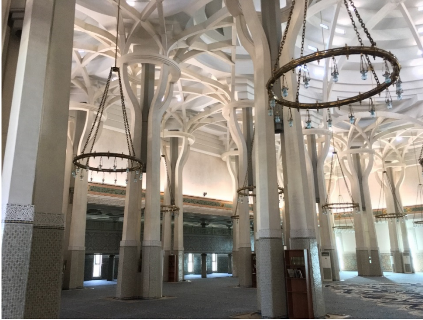
Fig. 29 - Interior concrete sculptural ceiling
