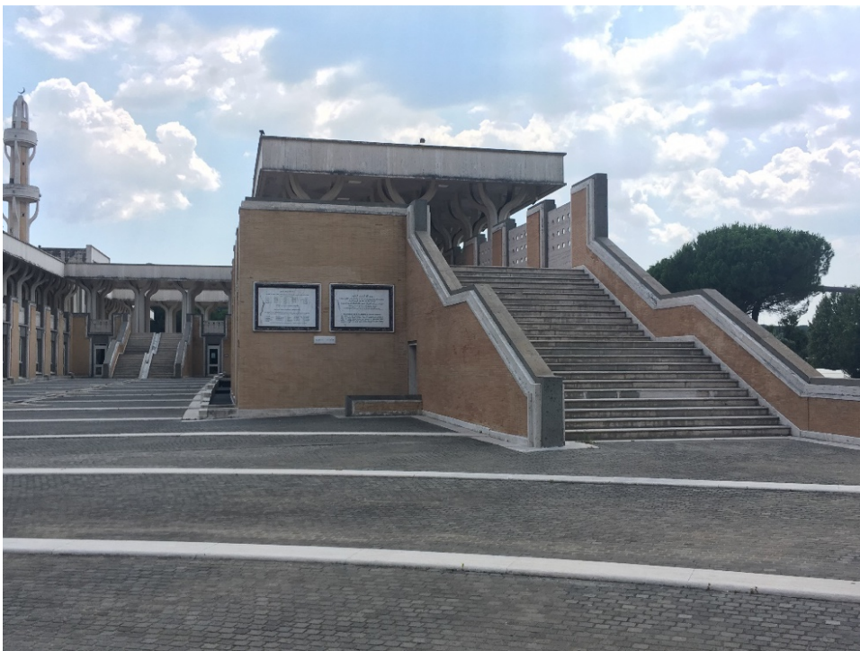
Fig. 36 - Built up levels forming ziggurat building shape
