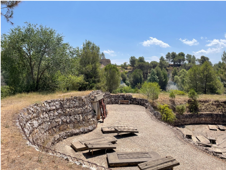
Fig. 10 - Cascade of earthworks
