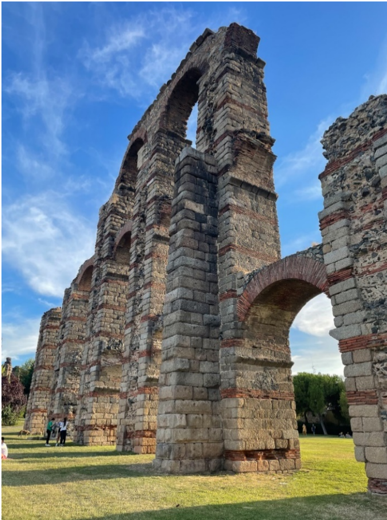
Fig. 5 - Brickwork arches and buttresses at aqueduct
