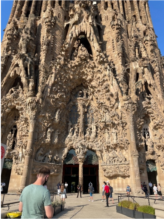
Fig. 33 - Parabolic arches in Nativity facade
