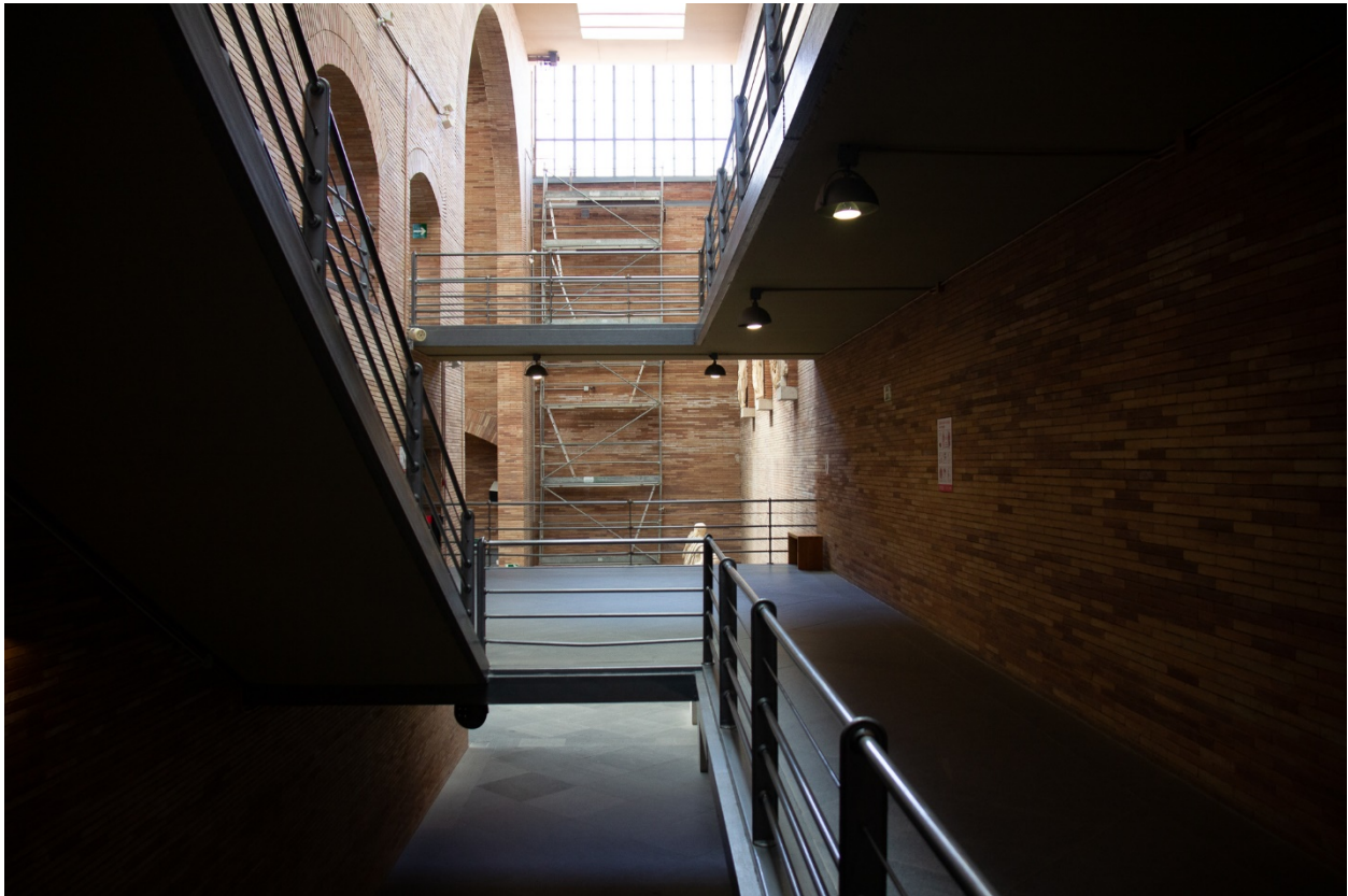
Fig. 26 - Brick bays and multi-level porous concrete walkways, with actual scaffolding for building repairs in background
