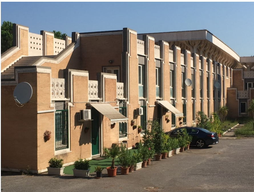
Fig. 28 - Travertine and brick cladding
