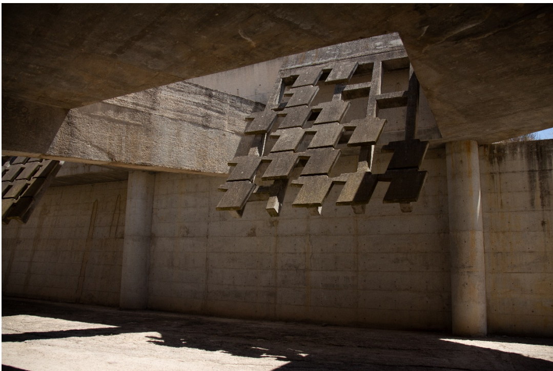
Fig. 29 - Dramatic falling ceiling planes
