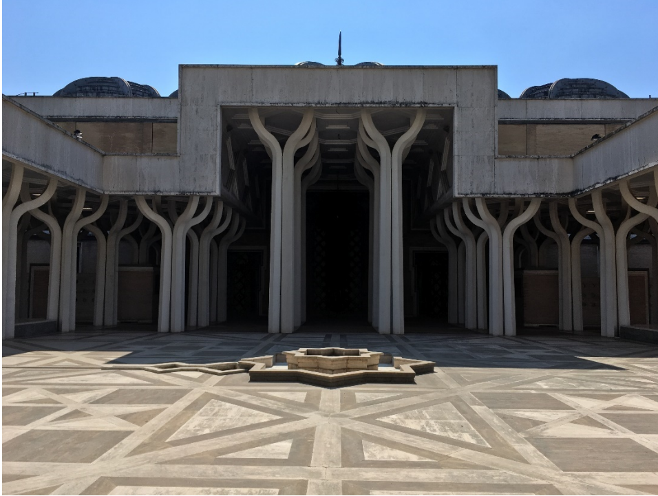
Fig. 19 - View of entry to prayer hall from more distant arcade and opposite side of courtyard. Visitors would come from entry arcade in the back left and unexpectedly find the large vestibule and entry.
