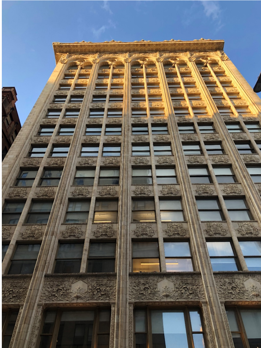
Fig. 3. Louis Sullivan, Details emphasize verticality, Bayard-Condict Building, New York City, New York, 1899.
