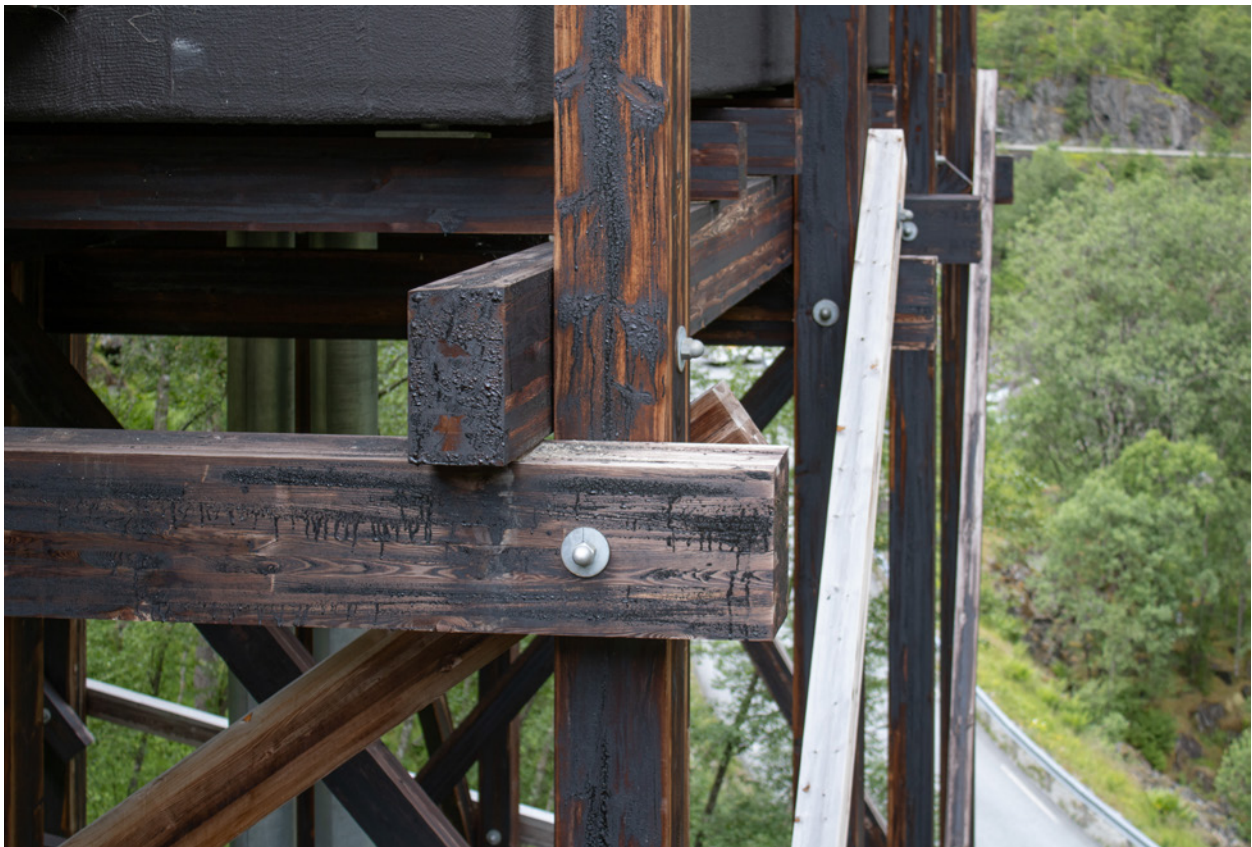
Fig. 23 Peter Zumthor, Creosote Timber Connections, Allmannajuvet Zinc Mine Museum, Sauda, Norway, 2016. Photograph by author.
