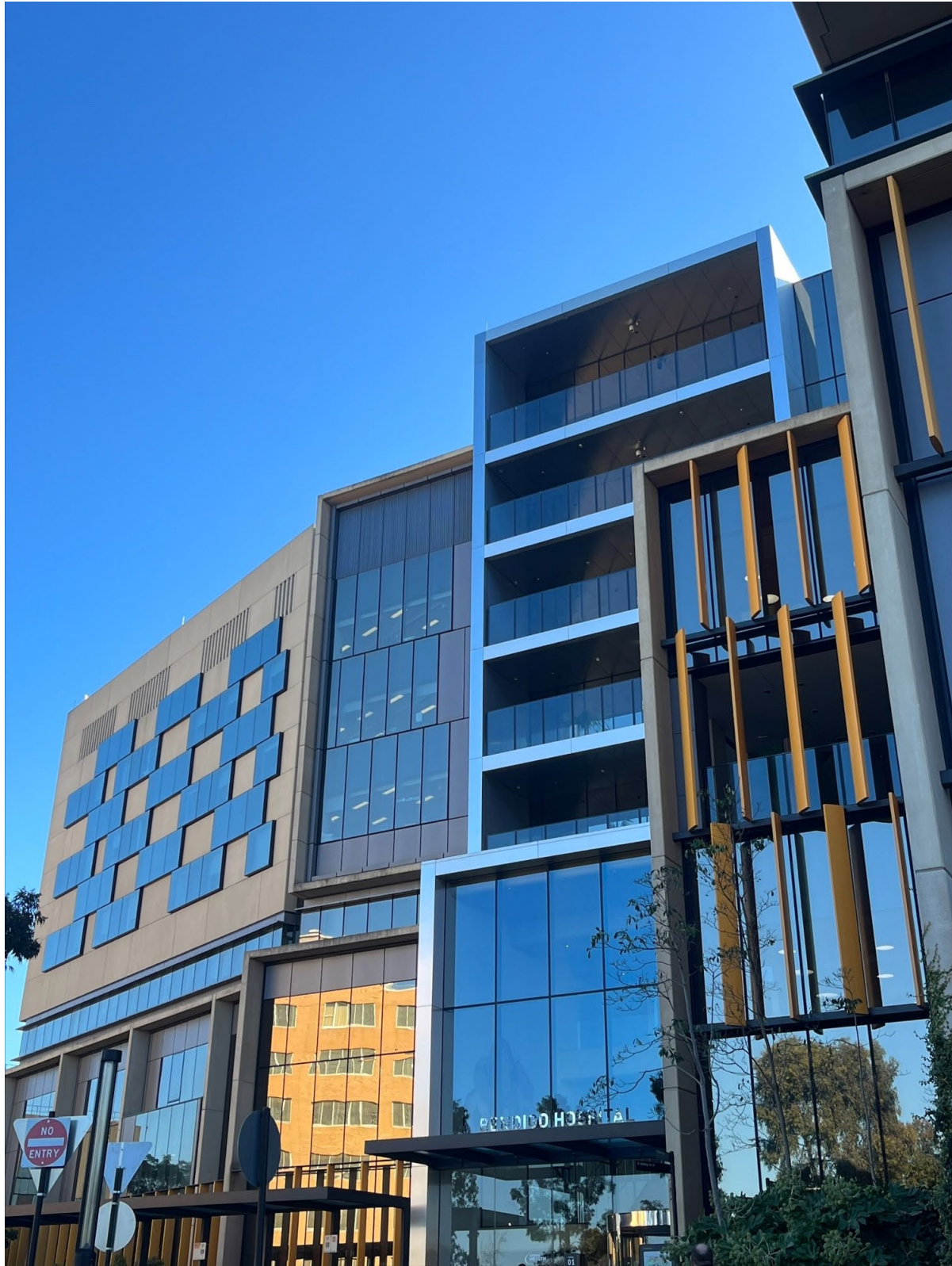
View from main entrance showing fragmented massing
