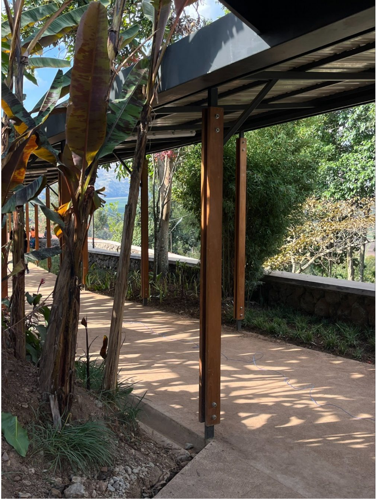
View of exterior hallway
