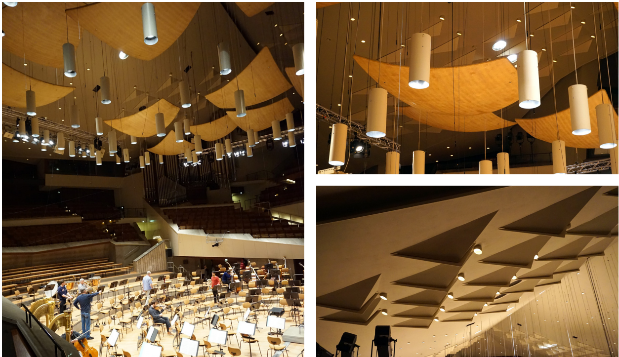
Fig. 12. Hans Scharoun. The acoustic elements of the hall ensure proper sound reflections and reverberation time. Berlin Philharmonic, Berlin, Germany, 1963.
