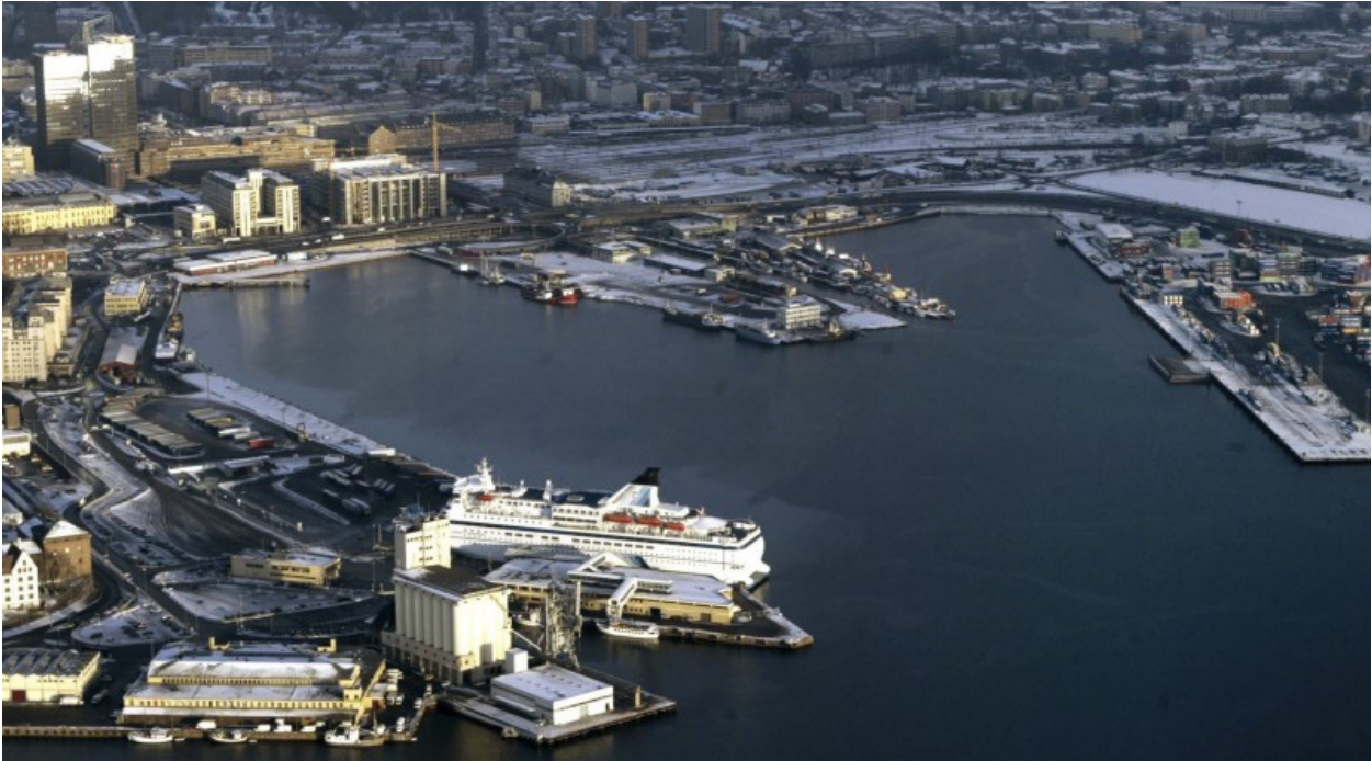
Fig. 2. Snøhetta. Aerial view of the site before construction began. Oslo Opera House, Oslo, Norway, 2008.
