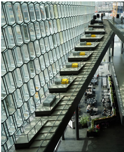
Fig. 7. Henning Larsen Architects. Tiered stair landings. Harpa Concert Hall, Reykjavik, Iceland, 2011.
