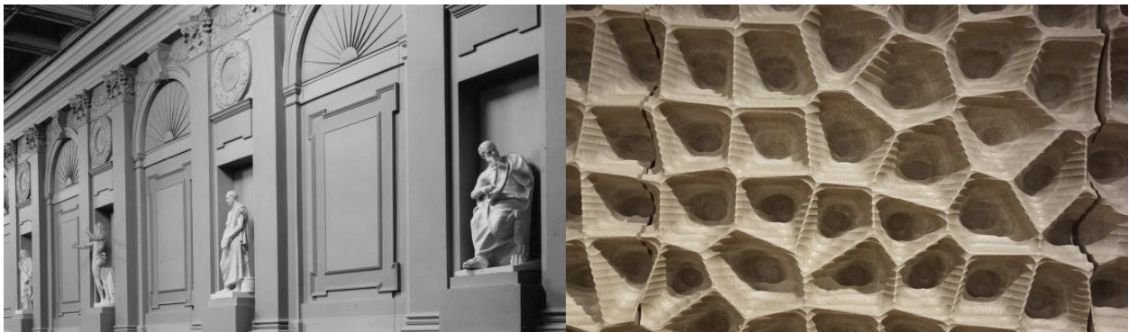
Fig. 15. Herzog and de Meuron. The milled gypsum panels achieve similar acoustic effects as plaster ornamentation used in 19th century concert halls such as Symphony Hall in Boston, MA. Elbphilharmonie, Hamburg, Germany, 2017.
