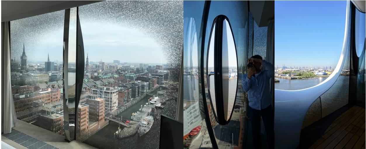
Fig. 18. Herzog and de Meuron. Variations on two curved glass forms allows for a dynamic facade, as well as places for operable windows and balconies. Elbphilharmonie, Hamburg, Germany, 2017.
